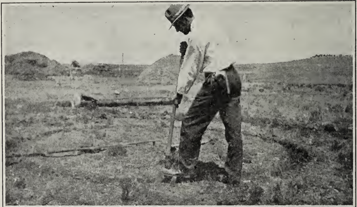
Fig. IV. County Agriculturist W. H. Lauck of El Paso county, helping build pit silos on farms in that county. Digging the trench for the concrete ring. Note the method of describing the circles. (Photo by Frear.)
