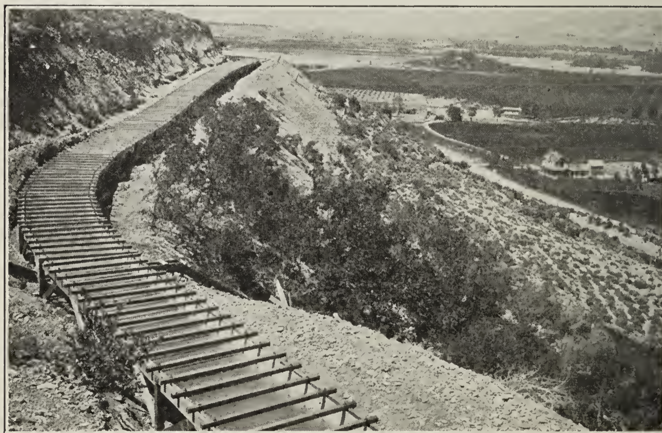
Plate II. Corrugated Flume, Stewart Canal, Paonia.
