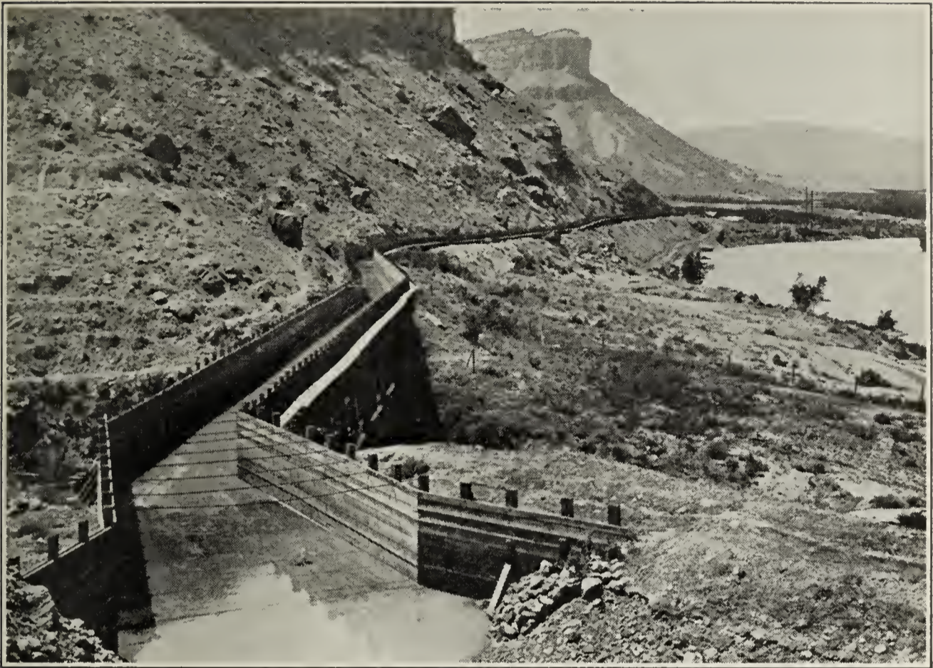
Plate III. Timber Flume, Orchard Mesa Power Canal, Palisade.
