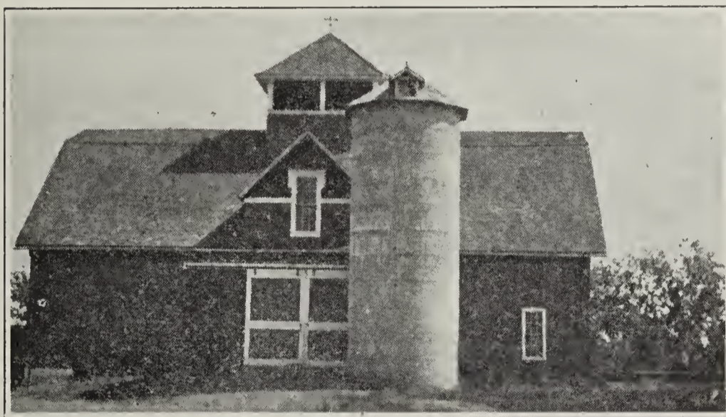
Dairy Barn and Concrete Silo, Colorado Agricultural College, Fort Collins
