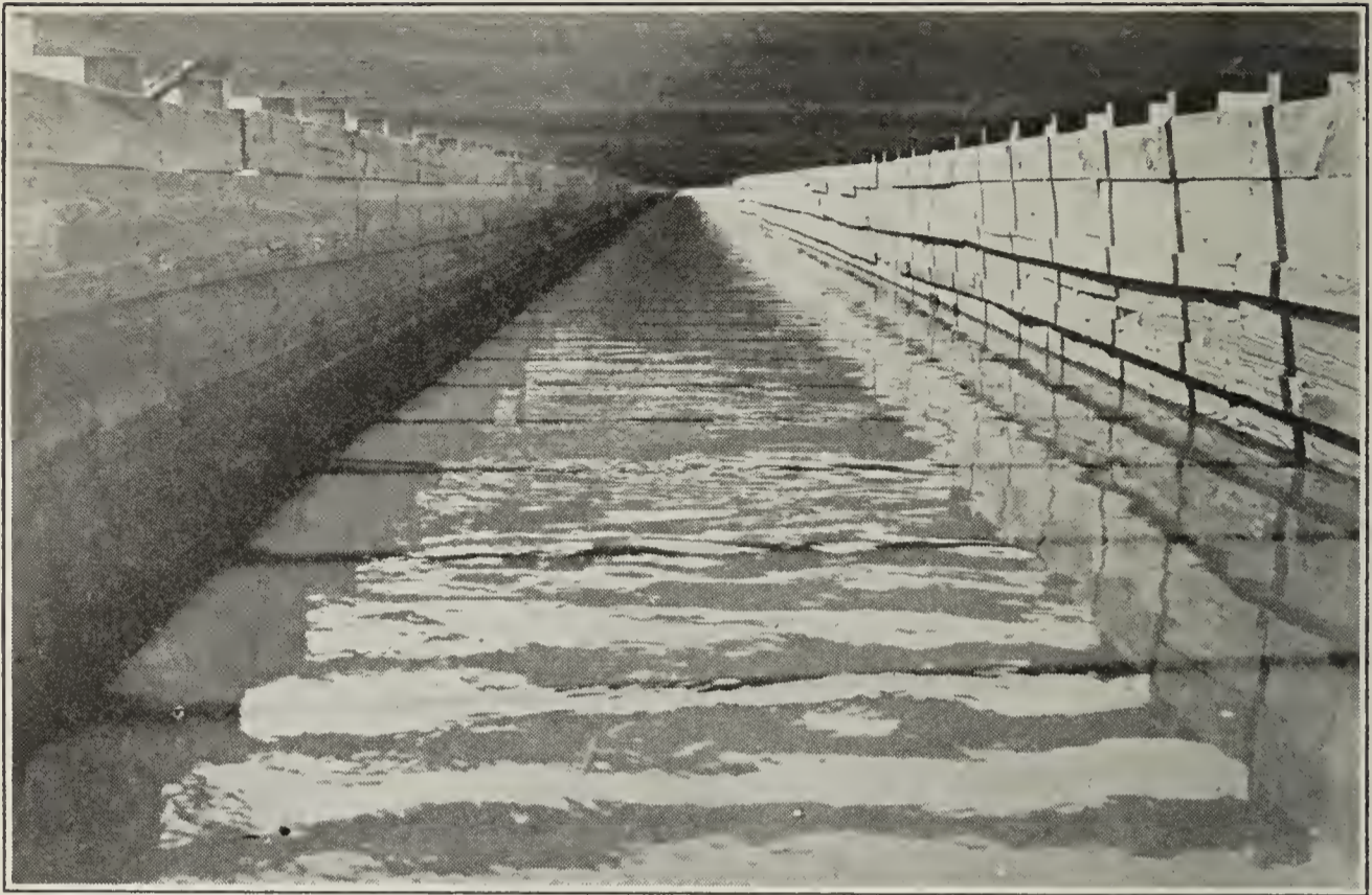
Plate V. Timber Flume Across Chicosa Creek, Fowler.
