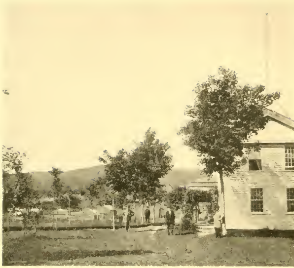
EAST END OF MOHICAN HOUSE. 1865
