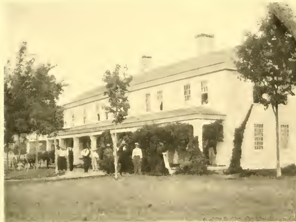
SOUTH SIDE OF MOHICAN HOUSE. 1865
