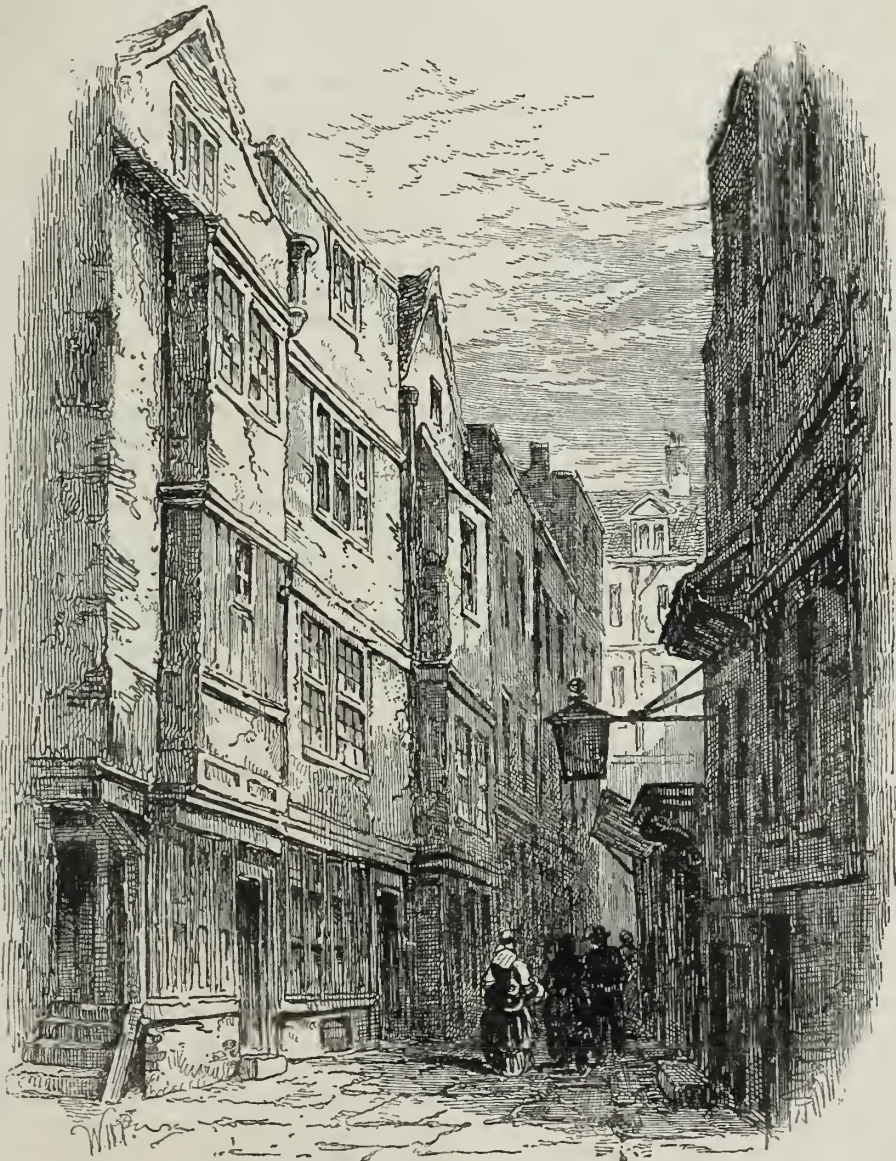
SERLE'S PLACE. From a Drawing taken shortly before its Demolition. (See page 21.)
