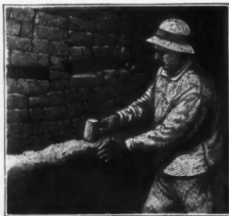
Showing man with which Plibrico is laid in place.
