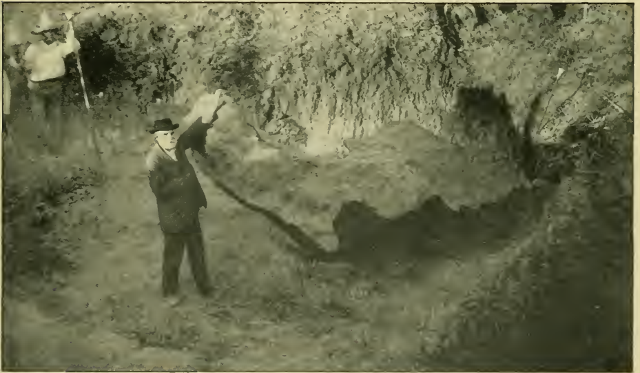
No. 2. AFTER FURTHER EXCAVATION.
