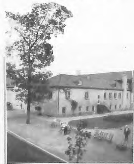
On the lower floor of this wing is the bakery. The kitchen department occupies the floor above it
