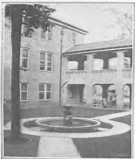
This was taken from the rear of the courtyard of the new cottage
