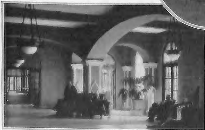
Here is a view of the lobby, looking toward dining-room and sun parlor. Above is the new dormitory cottage
