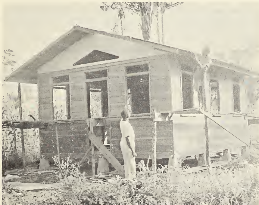
Figure 2.--A typical Surinam farmhouse under construction.
