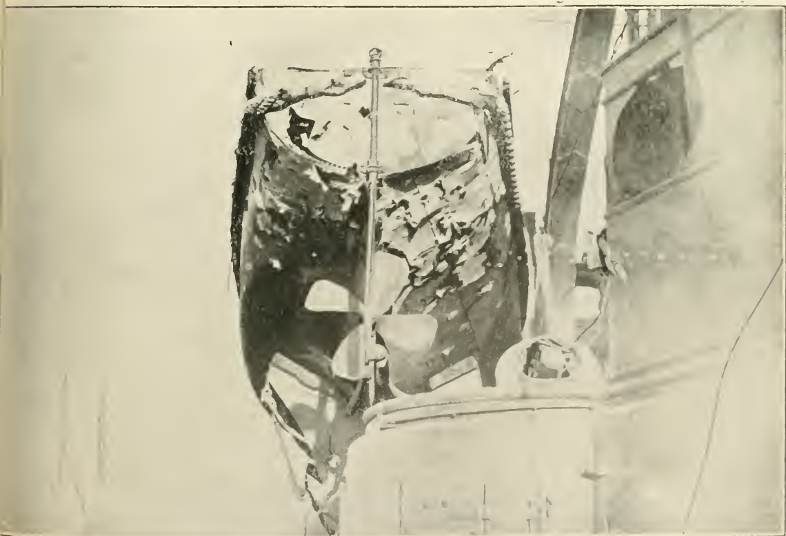
ONE OF THE "PALLADA'S" CUTTERS STRUCK BY A SHELL.
