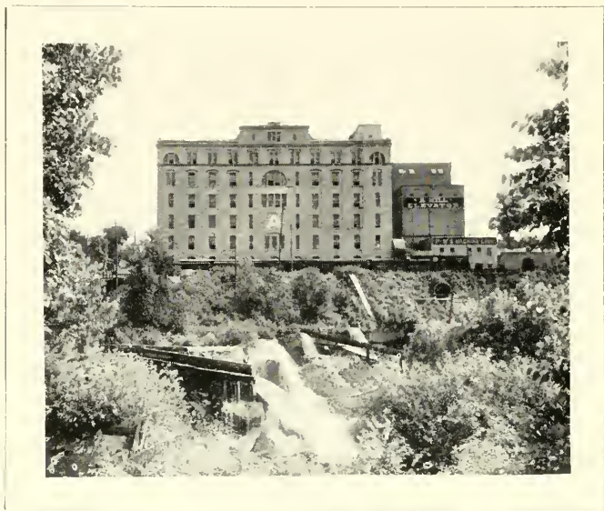
The "A" Mill Before the Erection of South "A"
