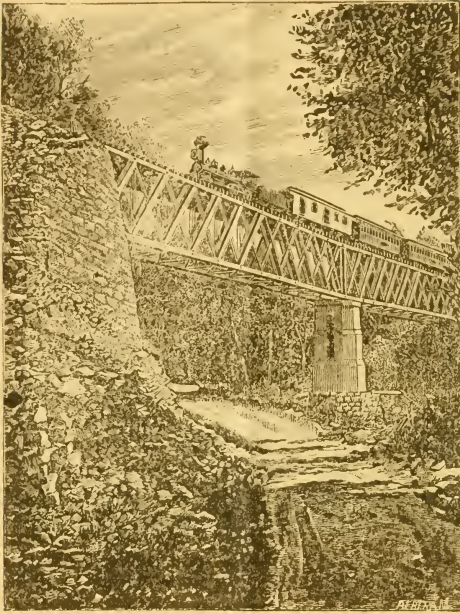
HIGH BRIDGE ABOVE MECHANICSTOWN.
