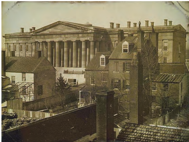
Figure 2. The Patent Office Building. This photograph was taken by John Plumbe about 1846 (Library of Congress, DAG No. 1229).
