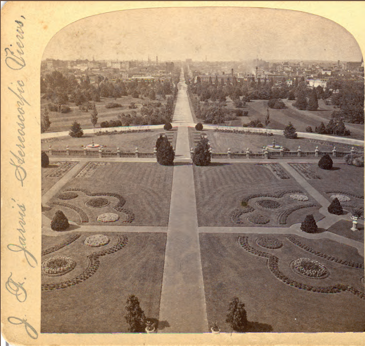
Figure 1. View looking north on 13th Street from the stairs of the Agriculture Building. This photograph was taken about 1880 (J.F. Jarvis' Stereoscopic Views, View from Agricultural Department, author's collection).
