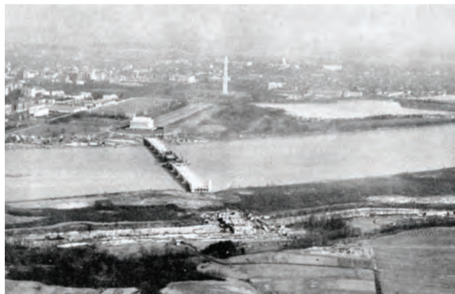
Figure 19. View looking north of the newly constructed Arlington Memorial Bridge directly connecting Arlington Experimental Farm with the National Mall. This photograph was taken about 1932 (author's collection).
