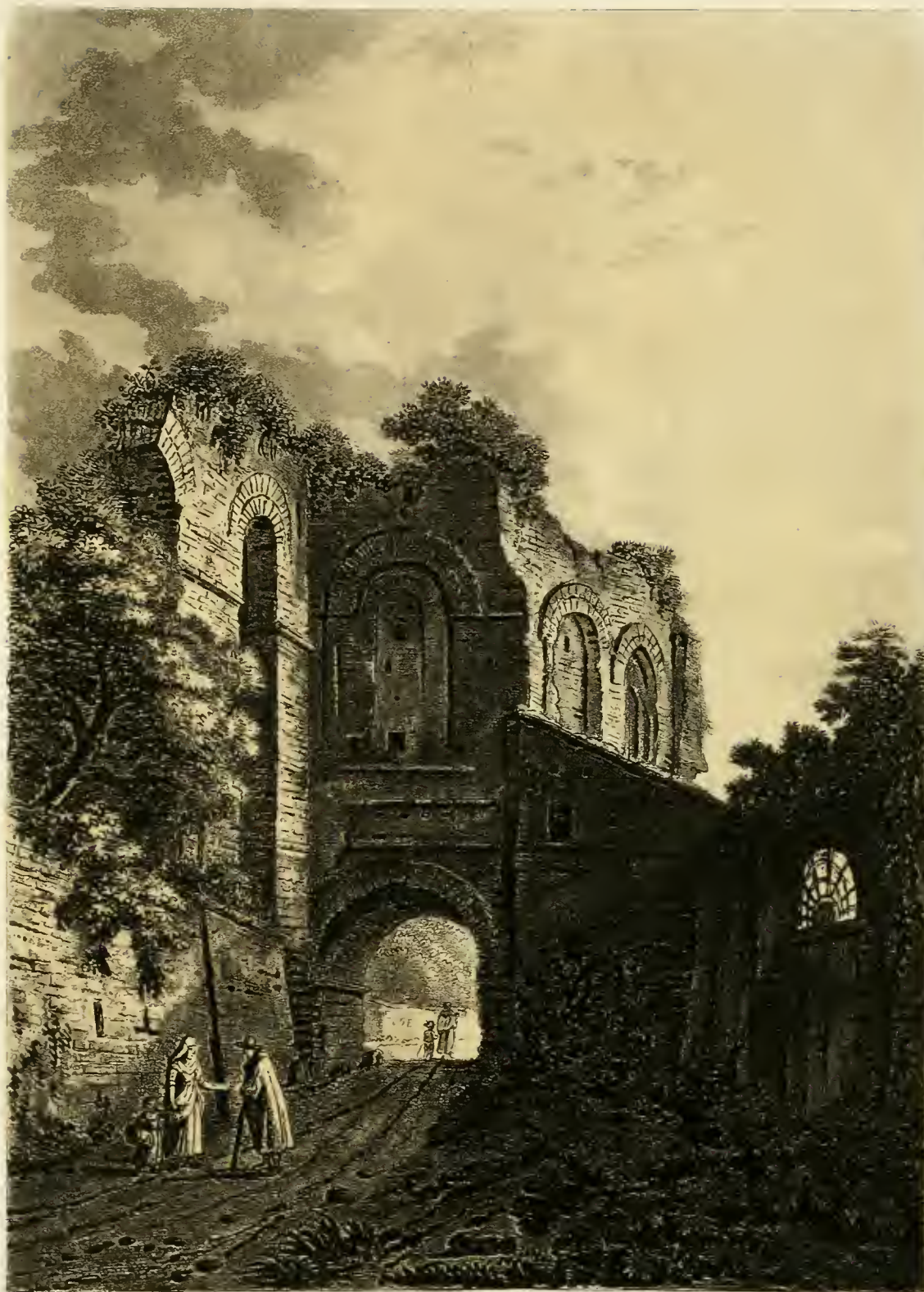
THE ARCH OF DOLABELLA.
