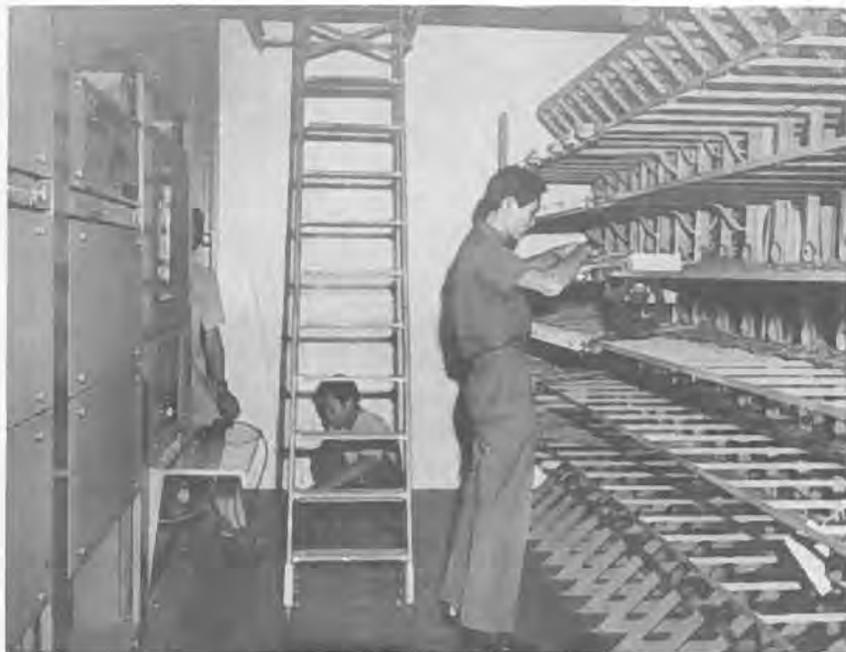
Telephone junction room
