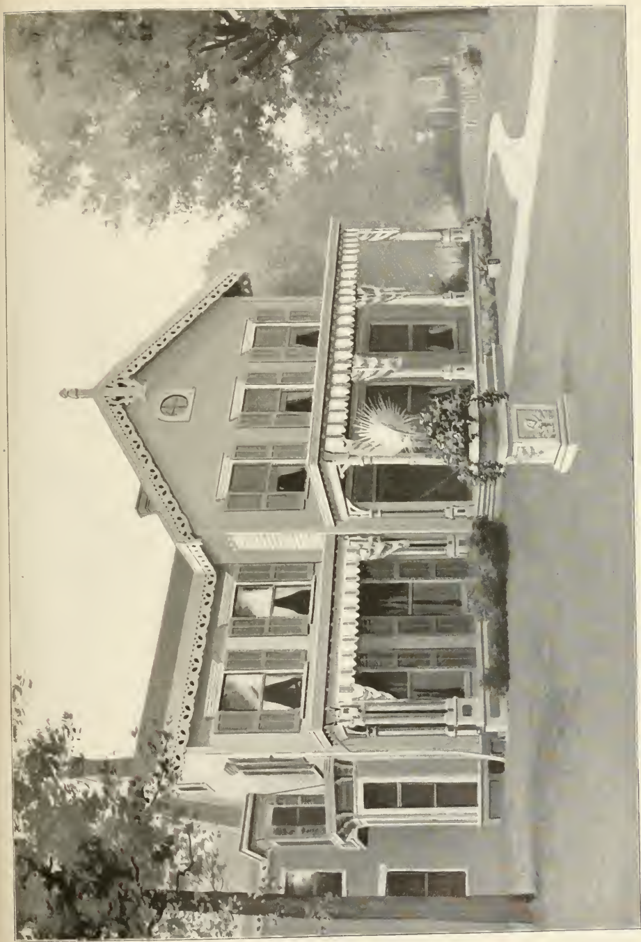
McKINLEY RESIDENCE, CANTON, OHIO
