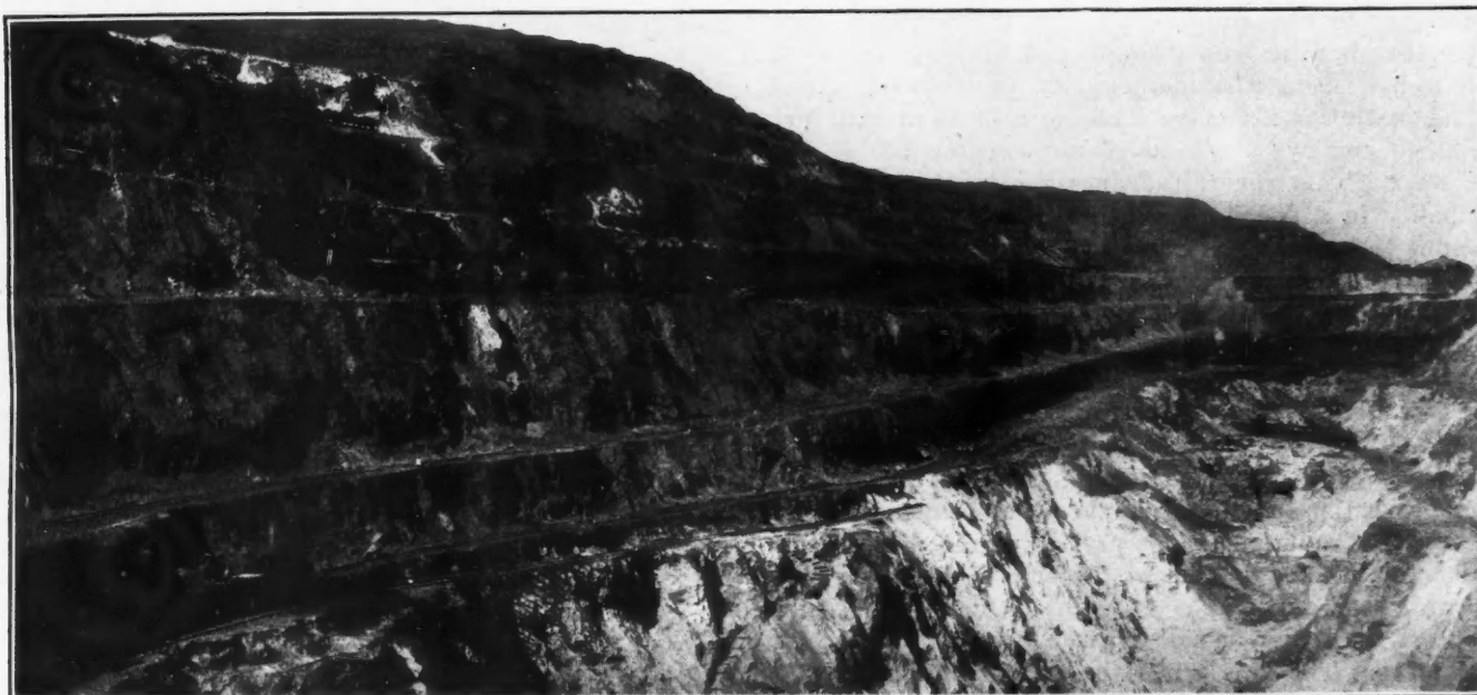
CORTA DEHESA, AT RIO TINTO, SHOWING TERRACED WORKINGS
