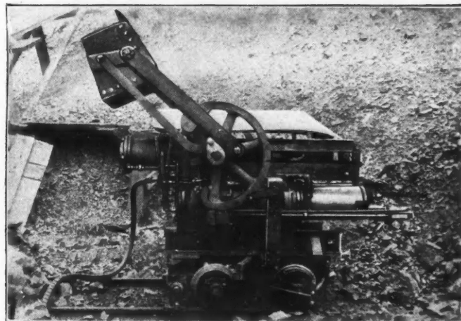
ARMSTRONG MECHANICAL ORE-LOADING SHOVEL
