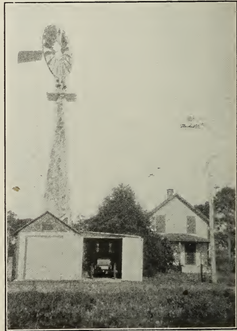
This is the windmill that turned the dynamo, that stored the batteries, of the electric auto (as it stands in its garage), that carried the potatoes to market.
