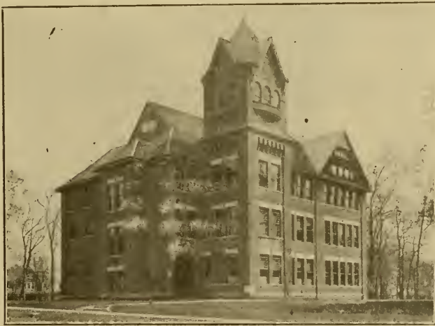
BURGESS MEMORIAL HALL.
