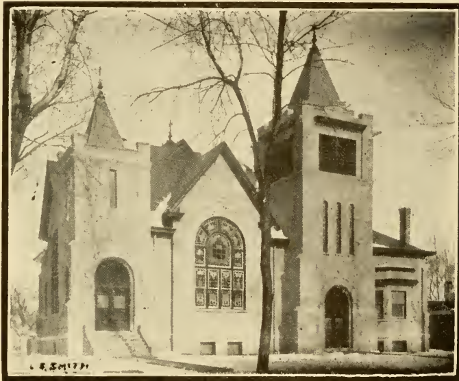
PRESBYTERIAN CHURCH, EL PASO, ILLINOIS.
