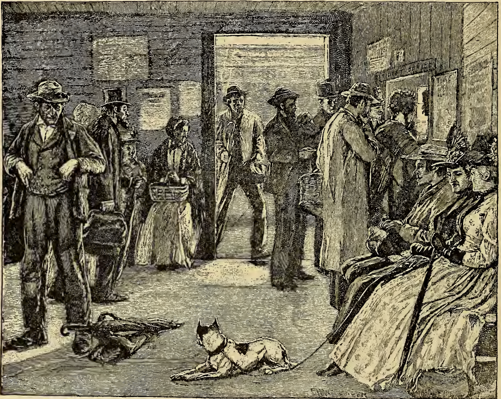
THE DEPOT AT SPRINGFIELD, ILLINOIS, FEBRUARY 11, 1861.
