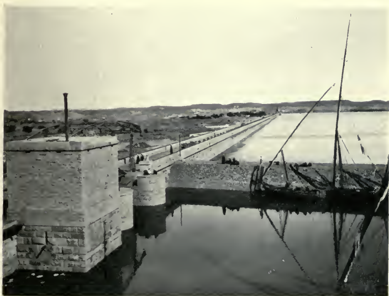
LOCK, BARRAGE AT ASSOUAN
