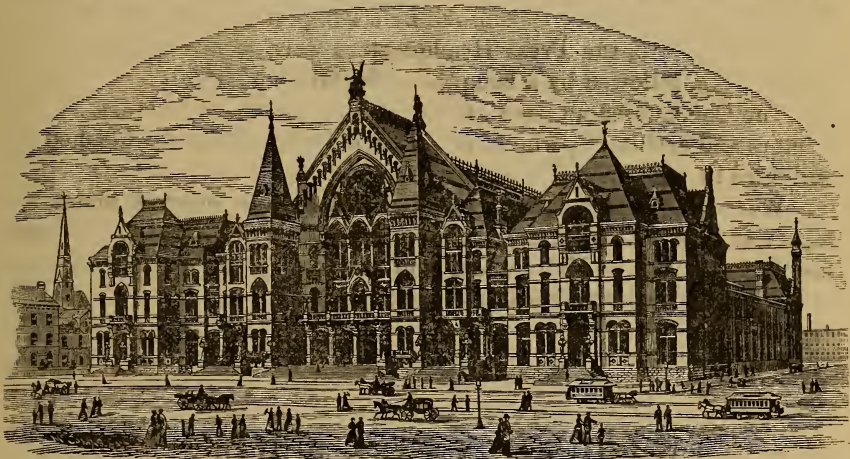
PERMANENT EXPOSITION BUILDINGS.
