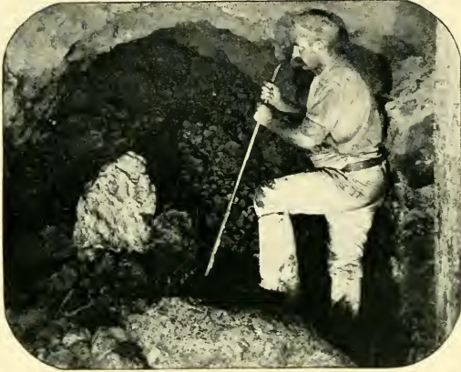
9.—De Beers Mine.—Underground Workings.
