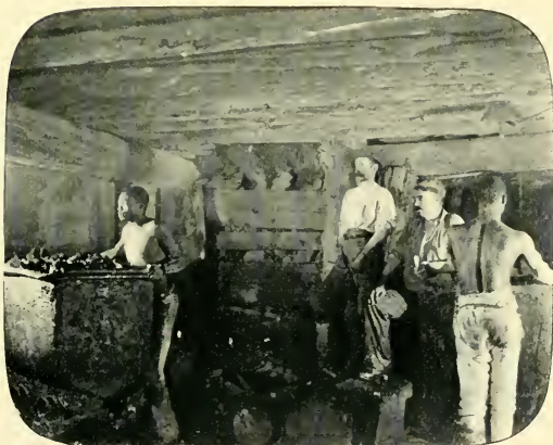
8.—De Beers Mine.—Underground Workings.
