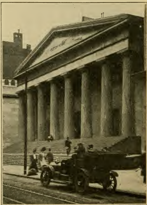
U. S. Custom House Chestnut between S. 4th and S. 5th Streets Page 56
