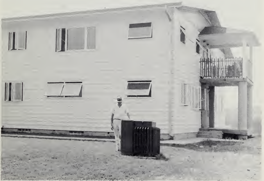
This prosperous Iowa farm requires more kwh than the 700 used by the average Linn County REC consumer. The 8-unit all electric apartment house (below) is a rare type of consumer on its lines. In front is 100-KVA single phase transformer, fed by an underground cable, which serves the building.
