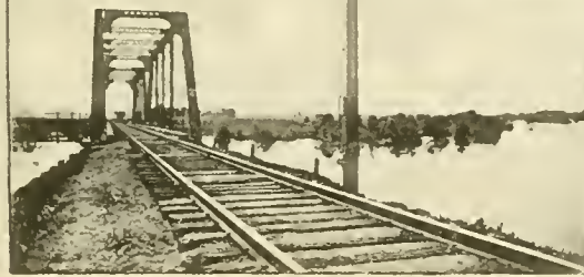
ILLINOIS CENTRAL RR BRIDGE ACROSS THE WAPSIPINICON
