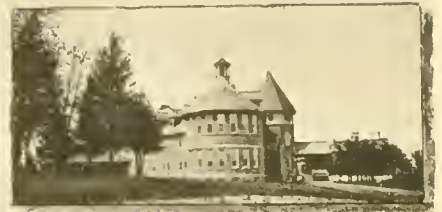
END VIEW WOMENS BUILDING
