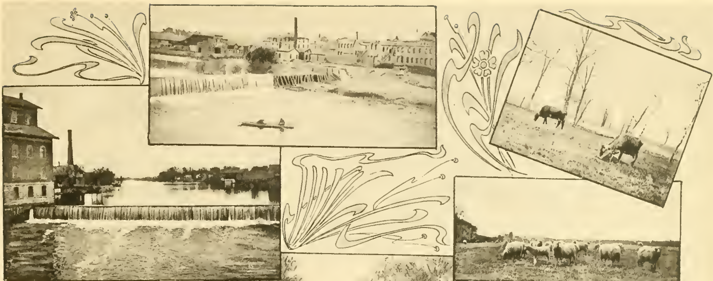
TWO VIEWS OF THE DAM.
