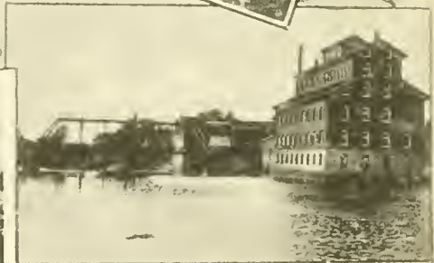
LOOKING SOUTH OVER THE DAM
