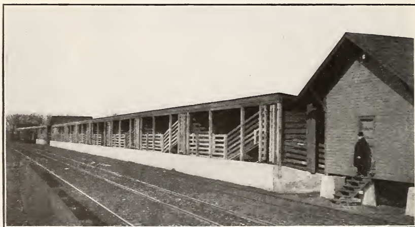
FIG. 2.—SAME YARD AS ABOVE AFTER RECONSTRUCTION.
