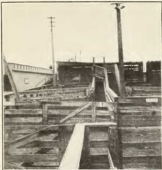
FIG. 1.—A GOOD UNLOADING CHUTE FOR DOUBLE-DECK CARS.
