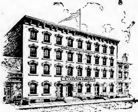
OCCUPYING THE ENTIRE BUILDING.
