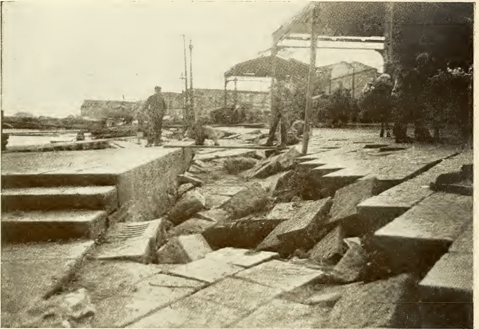
VIEW ALONG QUAY IN MESSINA SHOWING A DISPLACEMENT CAUSED BY LOCAL LAND-SLIPPING
