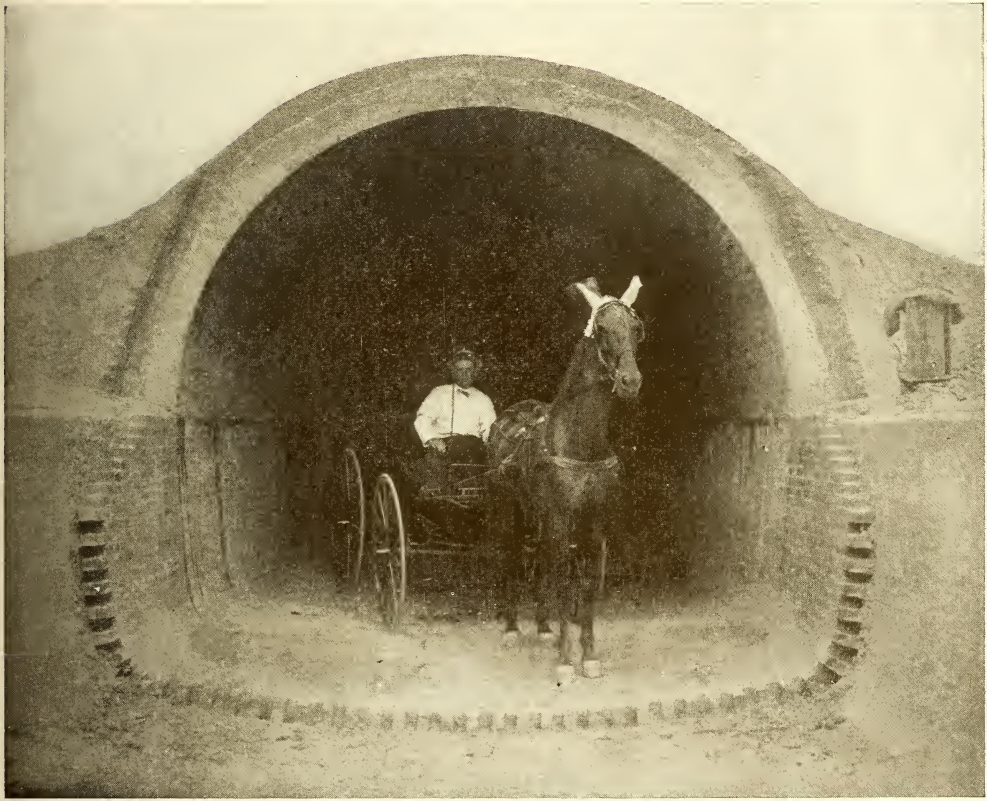
A COMPLETED SECTION OF THE OUTFALL SEWER
