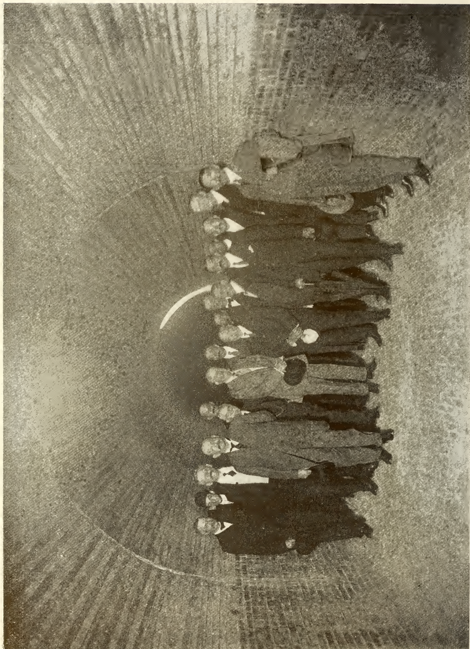
THE GOVERNOR OF MARYLAND, THE SEWERAGE COMMISSION, AND PARTY OF FINANCIERS ACCOMPANYING CHIEF ENGINEER HENDRICK ON A TOUR OF INSPECTION (VIEW TAKEN IN OUTFALL SEWER)
