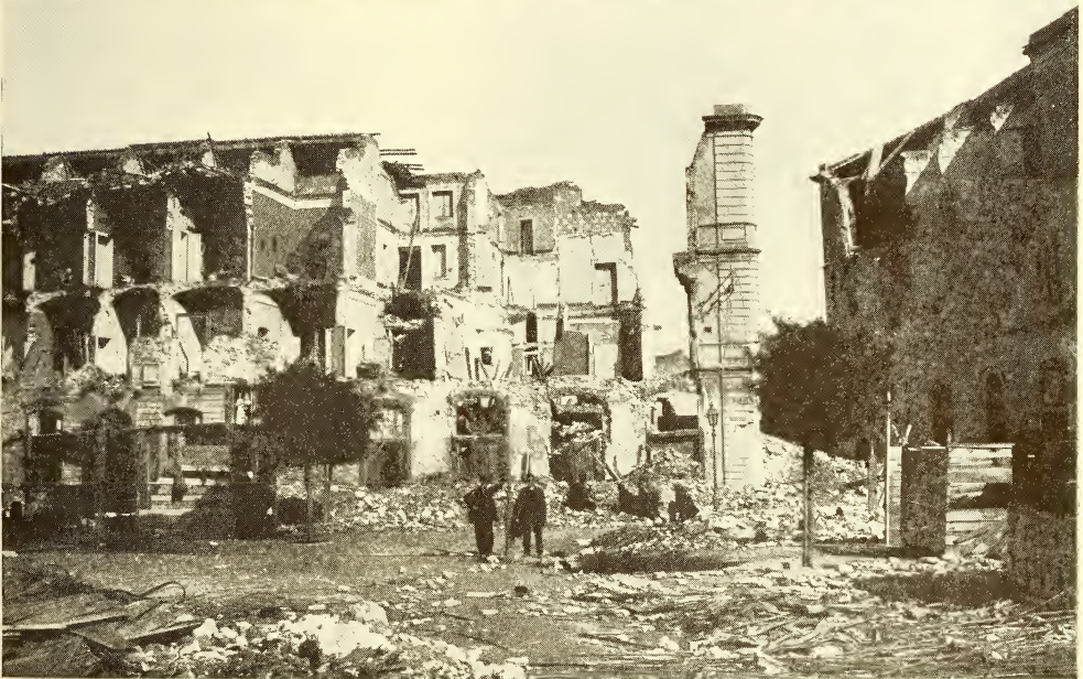
A FACTORY JUST SOUTH OF MESSINA The top of the chimney was thrown to the southeast
