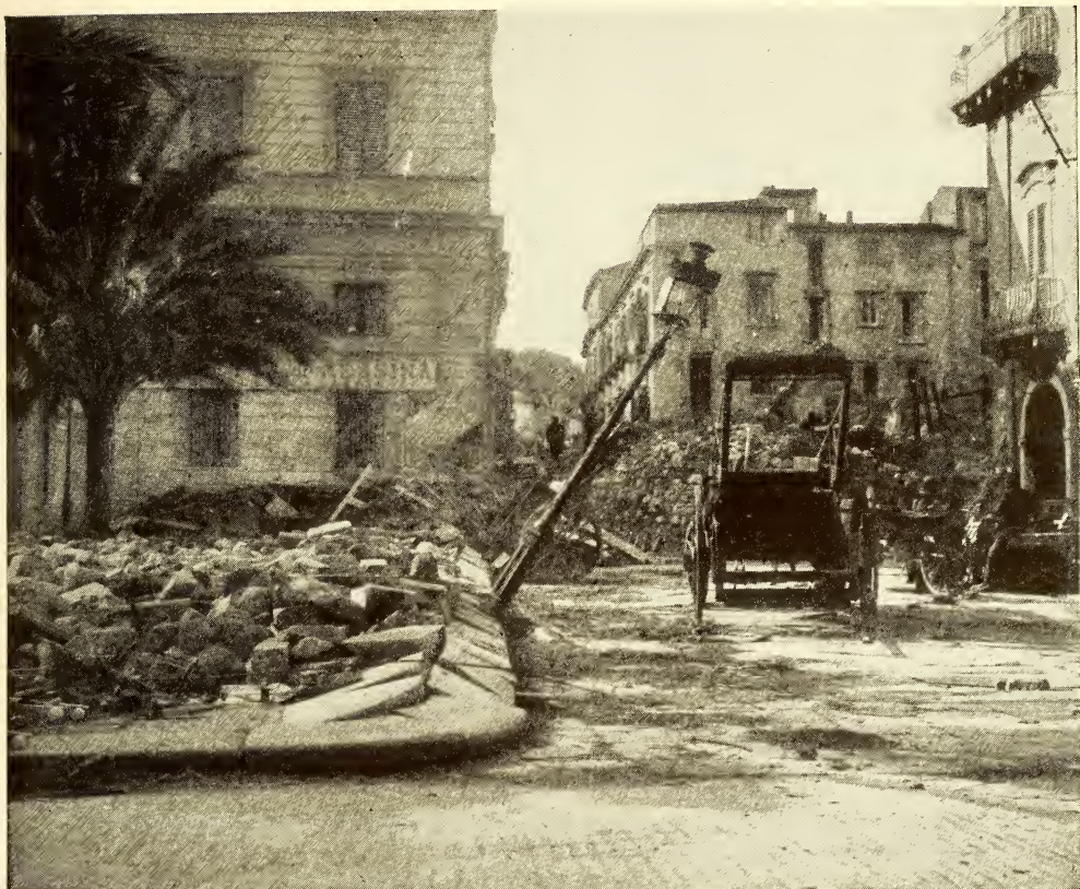
PIAZZA MUNICIPALI, SHOWING BUCKLING OF GRANITE BLOCKS CAUSED BY THE SEISMIC WAVE
