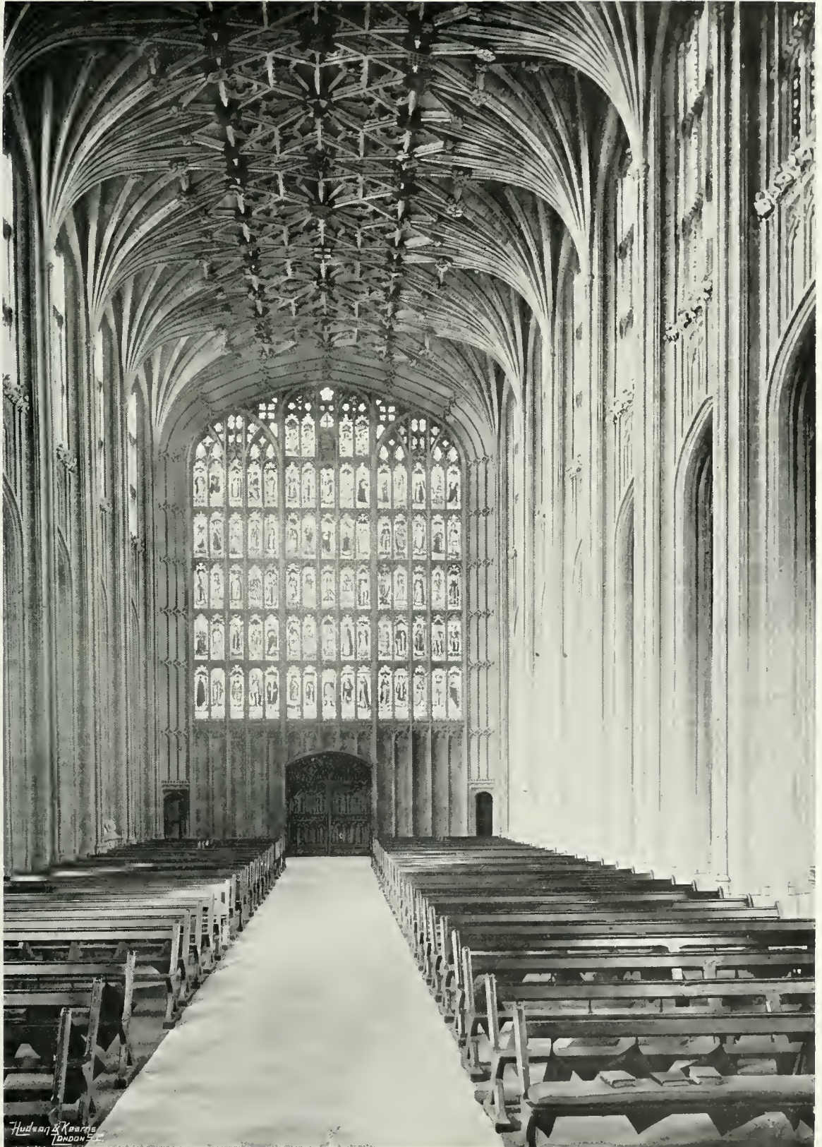
ST. GEORGE'S CHAPEL, THE NAVE, LOOKING WEST
