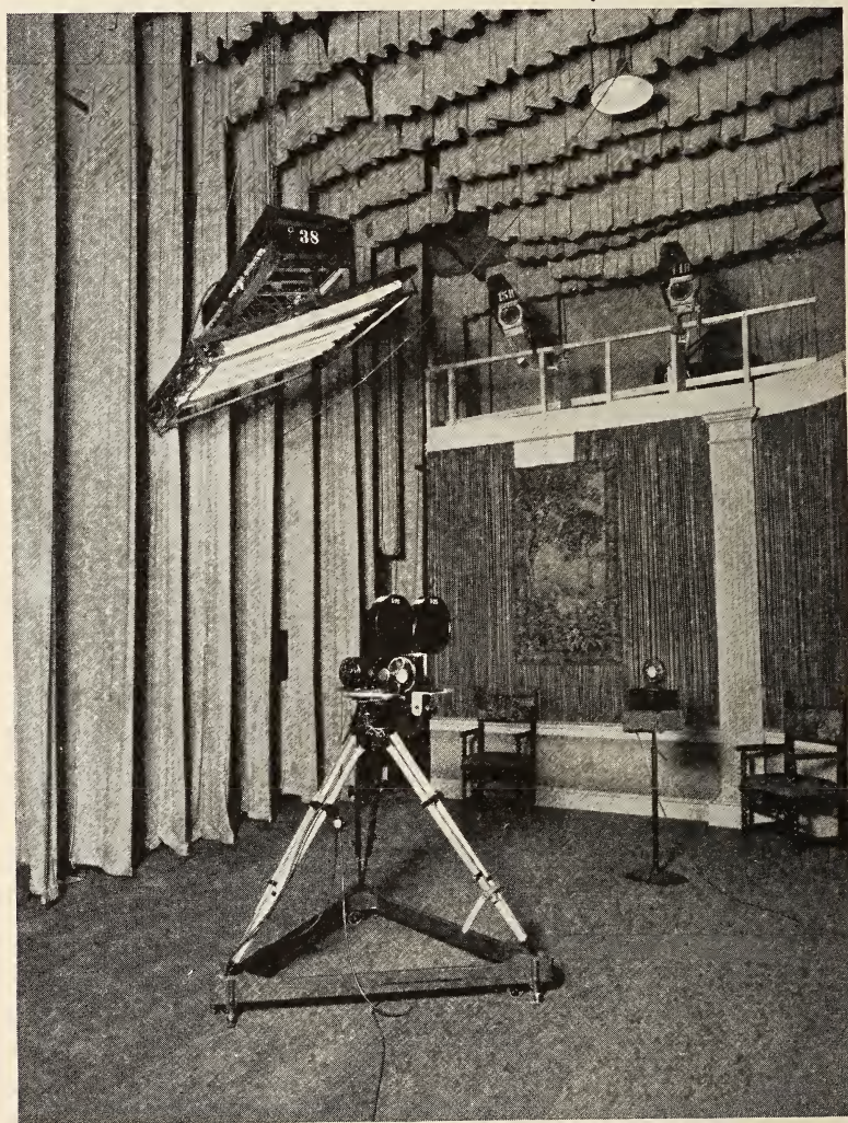
FIG. 1. Cloth drapes for controlling resonance in recording room.
