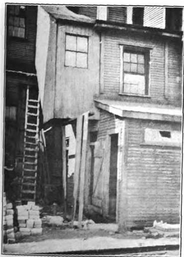
FIG. 40.—CLOSE-UP OF TWO-STORY TOILET. UPPER SECTION FOR WOMEN, LOWER FOR MEN. THIS TOILET IS A NUISANCE AND A HEALTH HAZARD.
