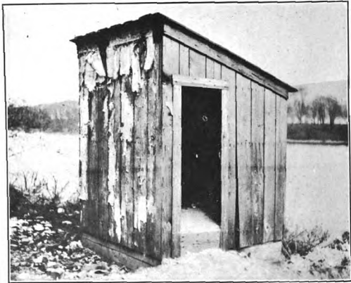
FIG. 37.—OUTDOOR PRIVY FOR MEN, CONTAMINATING STREAM OF WATER.
