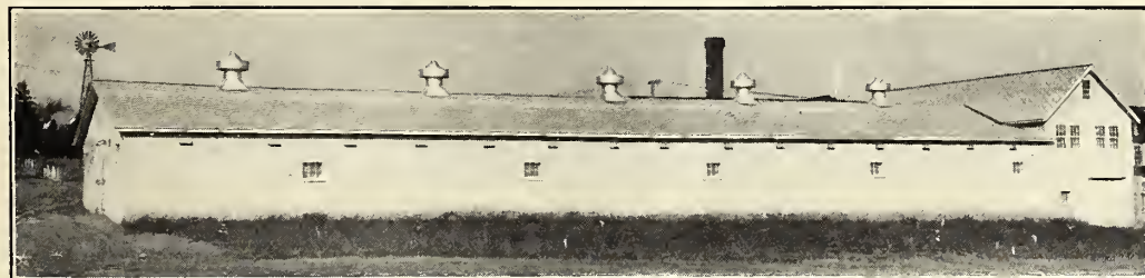
This new storage cellar provides for an additional hundred thousand Roses
