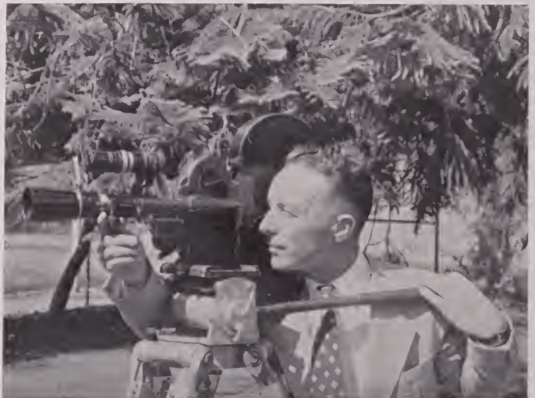
Joseph Yolo and the Eyemo Camera he has equipped with interlocked range finder.
