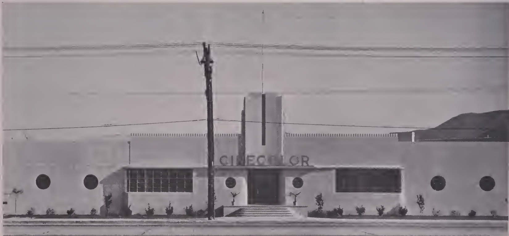
Front elevation of Cinecolor Laboratory in Burbank.
