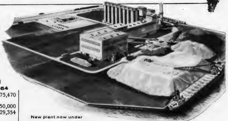
New plant now under construction in Milwaukee
