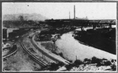
Bridge crossing Rio Grande Texas to New Mexico
