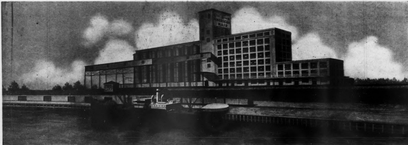
Plant of the AMERICAN MAID FLOUR MILLS, on the Houston Ship Channel
