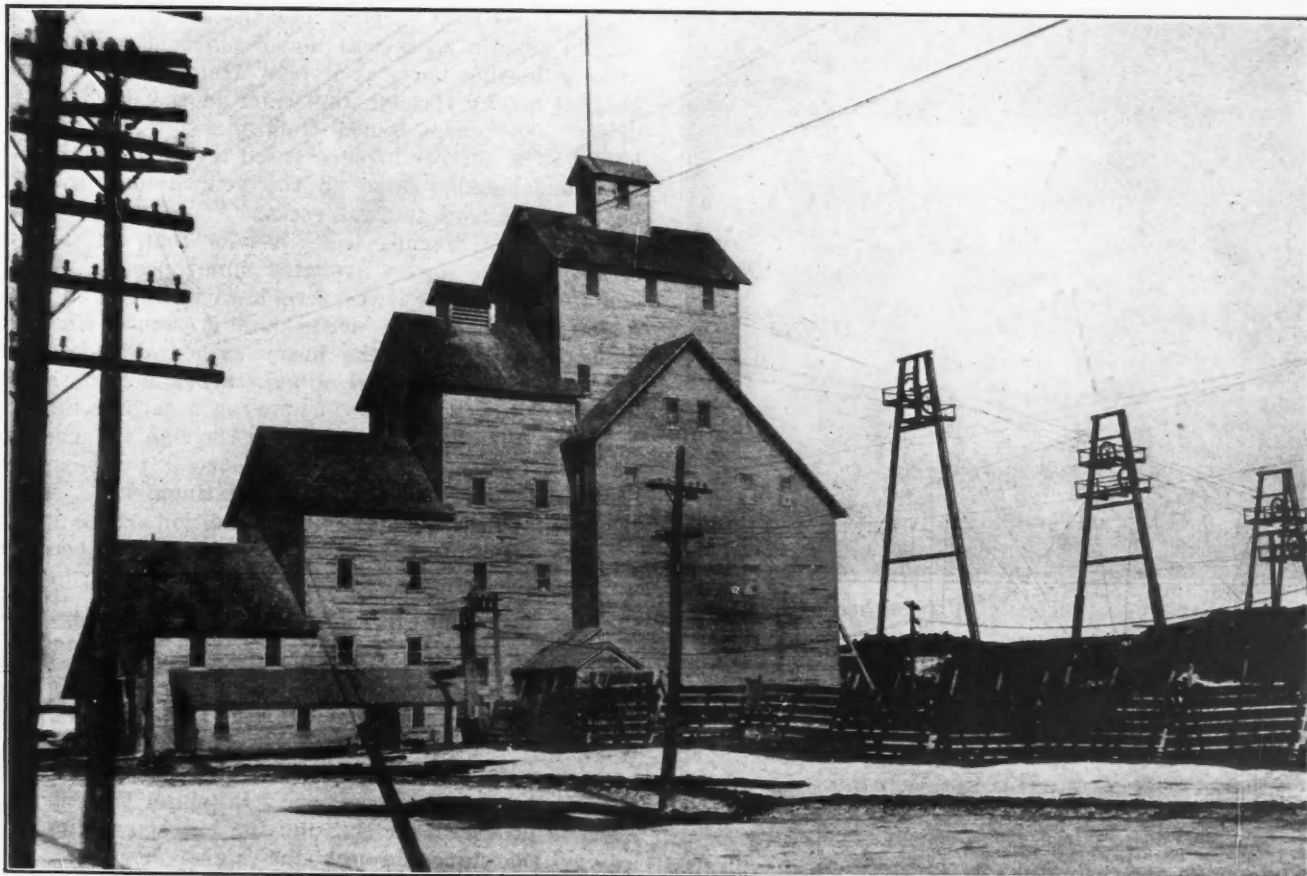
No. 6 hoist house of the Quincy Mining Co., Quincy, Mich.
