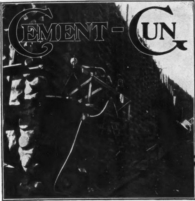
Protecting Cribbing—Hercules Mining Co.
