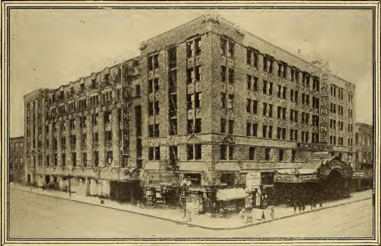
GRAUMAN'S METROPOLITAN THEATER, LOS ANGELES. ARCHITECT: EDWIN BERGSTROM. PLUMBING CONTRACTOR: J. HOKOM
