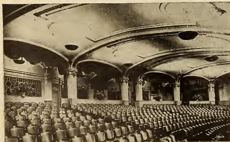
Night View Beneath the Balcony in a Medium Sized Motion Picture Theater, Totally indirect equipment is employed, a number of Mazda C lamps and mirrored glass reflectors being concealed by an ornamental composition housing. The location of outlets conforms with the decorative treatment of the ceiling. Soft, well diffused, glareless illumination is provided.
