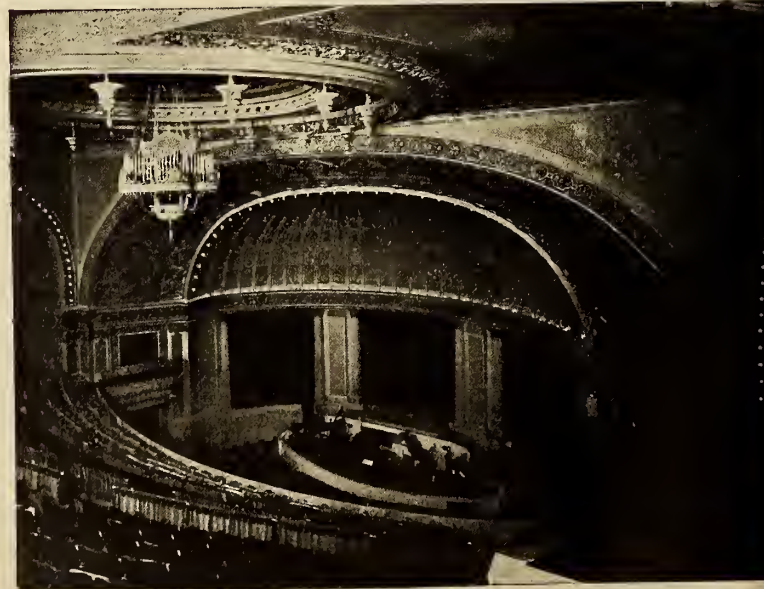
This View is Indicative of the Elaborateness of the Lighting Equipment in a Modern Motion Picture Theatre. The ceiling of the auditorium is of unusual beauty with a great dome 54 ft. across in the center which is lighted by 200 concealed lamps of various colors. At the center is suspended a chandelier of solid bronze, weighing 2500 lbs., 20 ft. long with a spread of 12 ft. This is fitted with 220 candle type lamps. The outer ring of the dome is illuminated by 16 indirect luminaires of unique design. A portion of the proscenium arch is of glass illuminated from behind and furnishing colored lighting effects during the overture.
