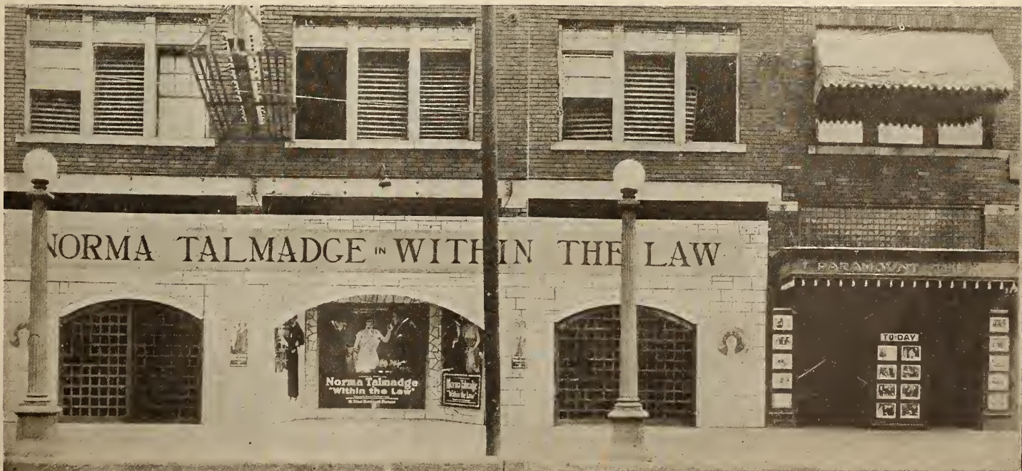
The Paramount Theatre, Logansport, Ind., has a lot of street frontage, and Manager William Lindsay makes use of every bit of it when he puts on displays for the big attractions, as shown by the arrangement above for First National's "Within the Law." With very little change in the arrangement of the compo board mask Mr. Lindsay had a colorful and appropriate setting for "The Bright Shawl," a bit of resourcefulness by which he proves that the small town house can afford to make displays.
