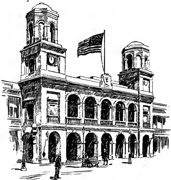
GOVERNMENT BUILDING, SAN JUAN.
