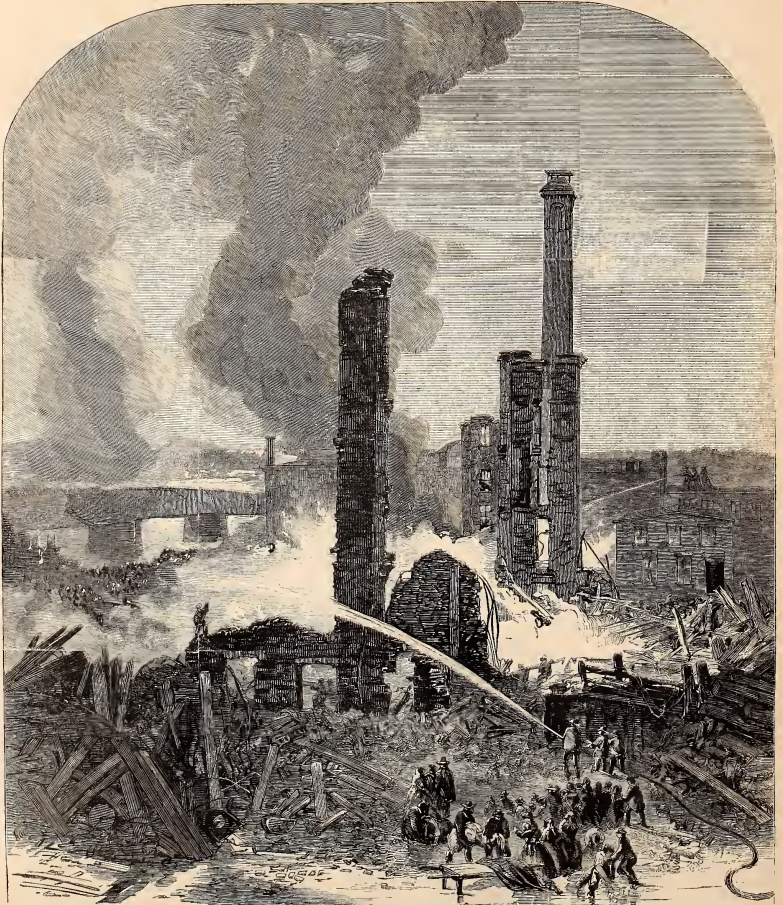
RUINS OF THE PEMBERTON MILLS, AT LAWRENCE, MASSACHUSETTS, THE MORNING AFTER THE FALL.—[FROM A PHOTOGRAPH BY WHISPLE, OF BOSTON.]
