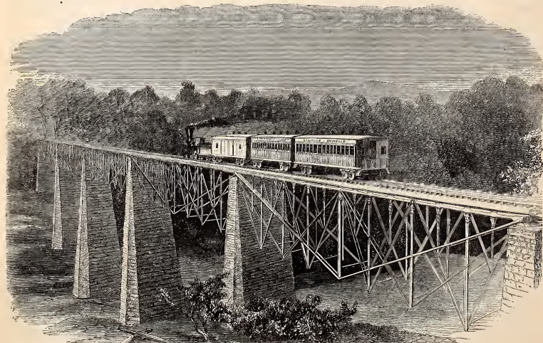
BRIDGE OVER GREEN RIVER, ON THE LOUISVILLE AND NASHVILLE RAILROAD.
