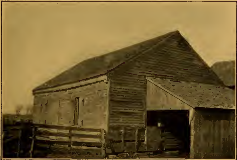
OLD LOG CHURCH, BUILT ABOUT SIXTY YEARS AGO The hewn logs are now covered with boards
