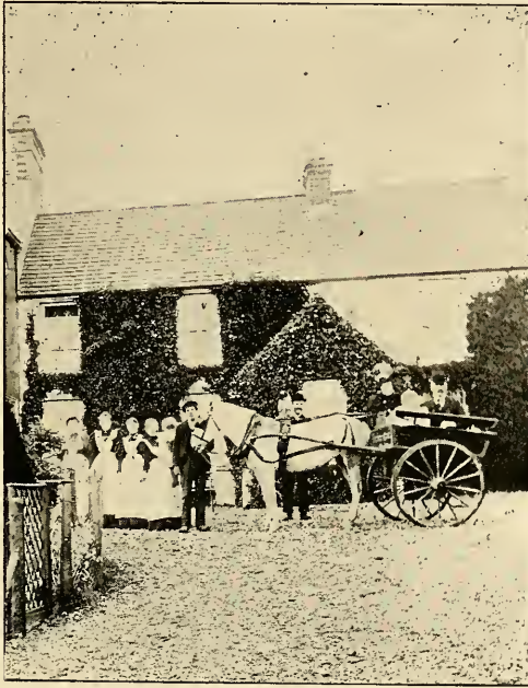
The window lowered from the top is of the room in which James Shields first saw light.
