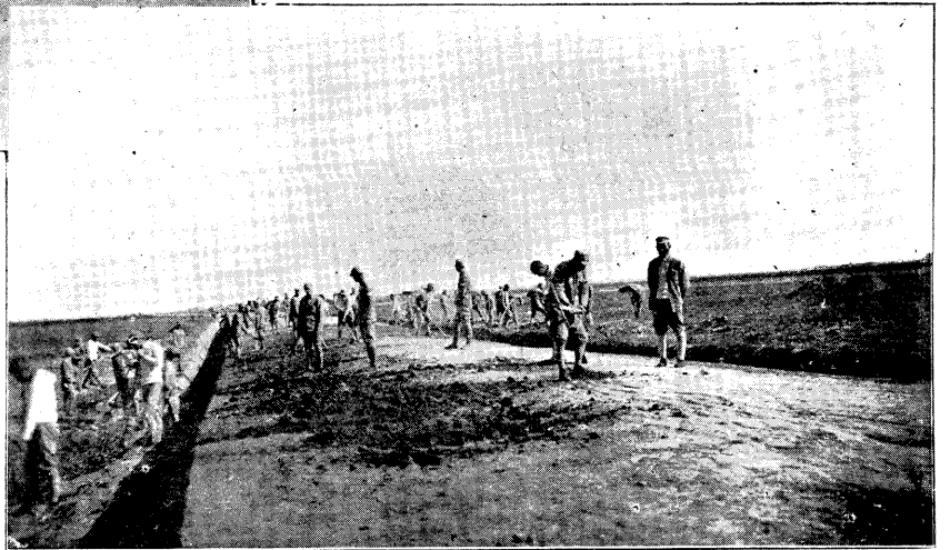
西蘭公路之兵工↑ SOLDIERS AT WORK ON THE SIAN-LANCHOW HIGHWAY
