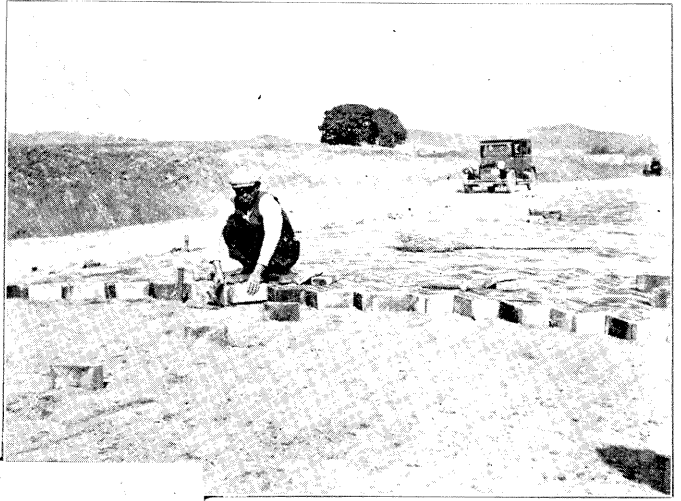
第一試驗路青磚路→ COMMON BRICK PAVEMENT ON THE FIRST EXPERIMENTAL ROAD
