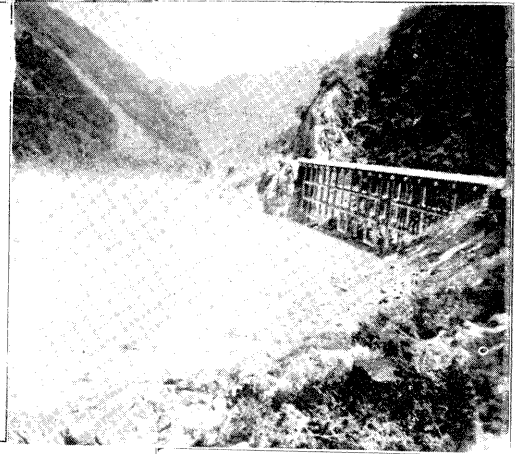
浙江縉麗路牛厄灘飛橋→ A REINFORCED CONCRETE TRESTLE BRIDGE ON THE TSINYUAN-LISHUI HIGHWAY IN CHEKIANG PROVINCE
