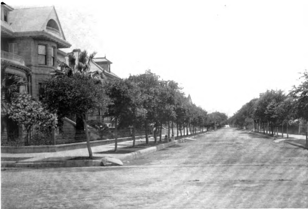
A TYPICAL RESIDENCE STREET IN THE RECONSTRUCTED CITY
