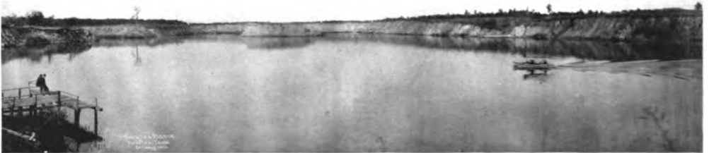
TURNING BASIN SHIP CHANNEL AT HOUSTON. "WHERE SEVENTEEN RAILROADS MEET THE SEA." EXCAVATIONS IN BACKGROUND SHOW LOCATION OF FREE MUNICIPAL WHARVES
