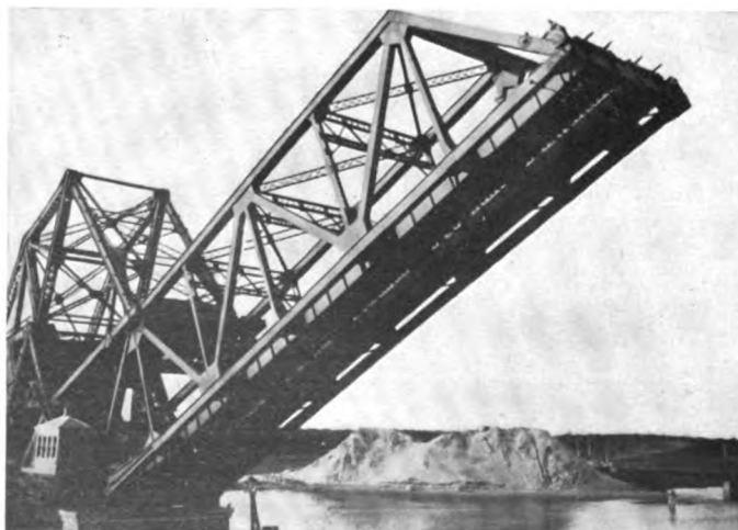
RAILROAD BRIDGE, HALF OPEN
