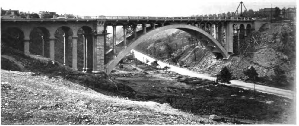
LARIMER AVENUE BRIDGE SPANNING THE BEECHWOOD BOULEVARD
