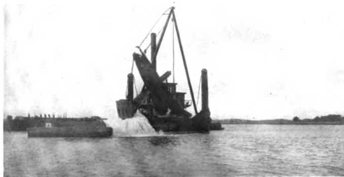
THE DREDGE "GOVERNOR WARFIELD" DIGGING THE CANAL AT THE RATE OF 10 CUBIC YARDS PER BITE.
