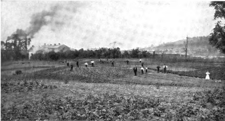
BRIDGE BUILDERS TENDING THEIR GARDENS IN OFF HOURS
