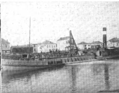
UNDAUNTED BY DISASTER, HER CITIZENS VALIANTLY UNDERTOOK AND BRILLIANTLY ACCOMPLISHED THE STUPENDOUS TASK OF PLACING GALVESTON PERMANENTLY ABOVE FLOOD LEVEL. HUGE SUCTION DREDGES CARRIED SAND FILLING INTO THE CITY AND EVERY HOUSE WAS RAISED SO AS TO BE EXACTLY ON THE GROUND WHEN THE FILLING WAS COMPLETED
