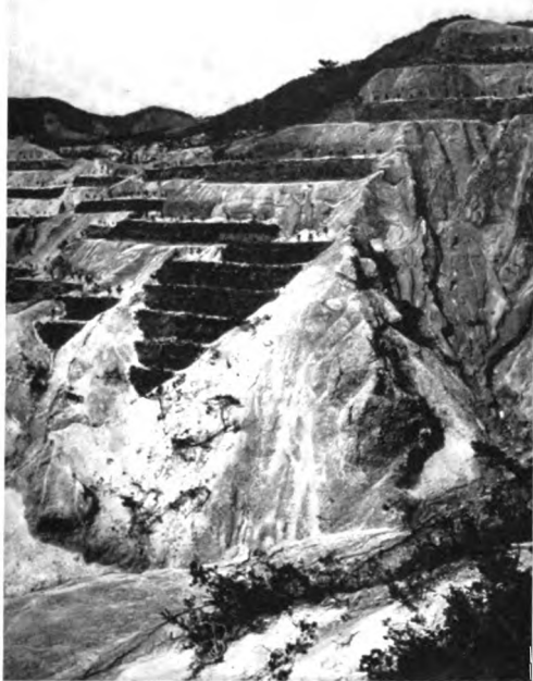
THAT THE JAPANESE ARE NOT AFRAID TO ATTACK A HARD PROBLEM IS SHOWN BY THIS ILLUSTRATION OF THE TERRACING AND TURFING CARRIED OUT IN HIROSHIMA, JAPAN, AS THE FIRST STEPS TOWARD REFORESTING A STEEP AND BADLY ERODED MOUNTAIN SIDE
