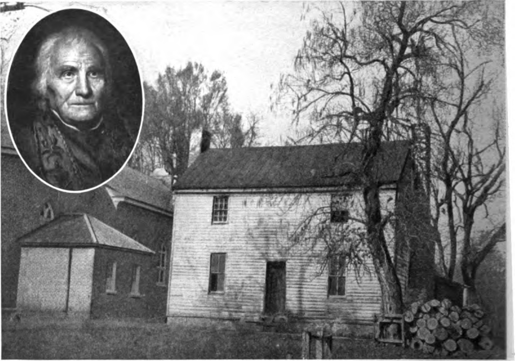
THE OLD EPISCOPAL RESIDENCE AT BARDSTOWN, KY.
