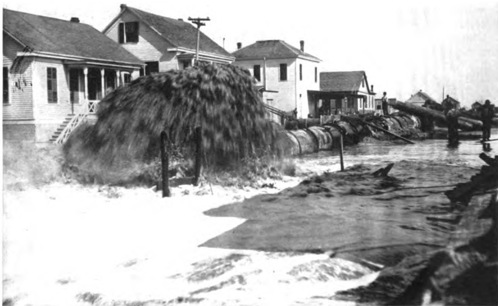
THE WATER RAN OFF AND THE SAND REMAINED
