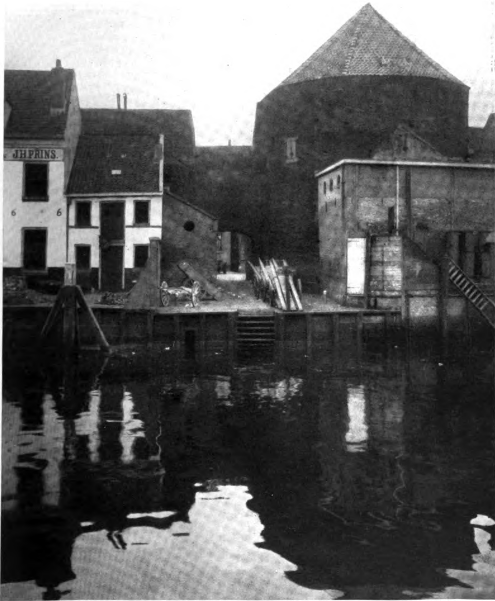
THE PEISTERPOORTGE, AND ALL THAT REMAINS OF ZWOLLE'S OLD WALLS
