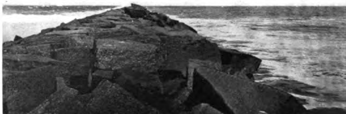
A GLIMPSE OF THE GREAT STONE BREAKWATER, EXTENDING 3000 FEET INTO BARNSTABLE BAY, WHICH PROTECTS THE NORTHERLY ENTRANCE TO THE CAPE COD CANAL.
