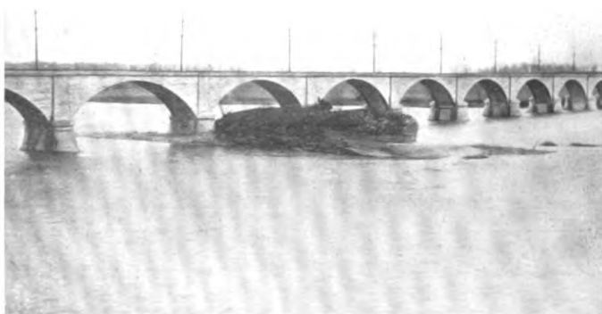
CONCRETE ELECTRIC RAILWAY BRIDGE SPANNING THE MAUMEE RIVER, BETWEEN WATERVILLE AND "ROCHE DE BOUT," NEAR TOLEDO, O.
