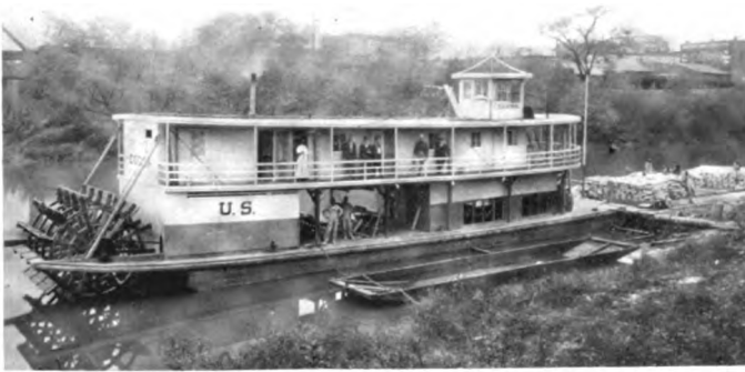
GOVERNMENT TUG USED IN WORK ON LOCK AND DAM AT MAYO'S BAR, EIGHT MILES BELOW ROME, GA.
