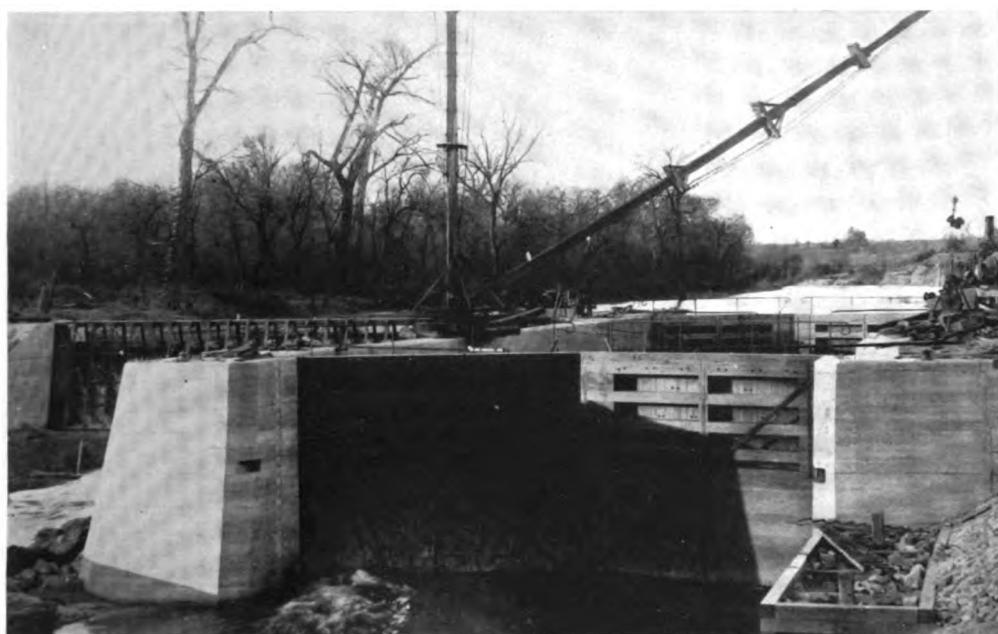
SCENE AT LOCK AND DAM NO. 1, THIRTEEN MILES BELOW DALLAS SHOWING IMPROVEMENT EFFECTED IN NAVIGATION OF BRAZOS RIVER
