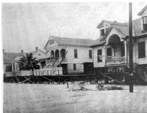
UNDAUNTED BY DISASTER, HER CITIZENS VALIANTLY UNDERTOOK AND BRILLIANTLY ACCOMPLISHED THE STUPENDOUS TASK OF PLACING GALVESTON PERMANENTLY ABOVE FLOOD LEVEL. HUGE SUCTION DREDGES CARRIED SAND FILLING INTO THE CITY AND EVERY HOUSE WAS RAISED SO AS TO BE EXACTLY ON THE GROUND WHEN THE FILLING WAS COMPLETED
