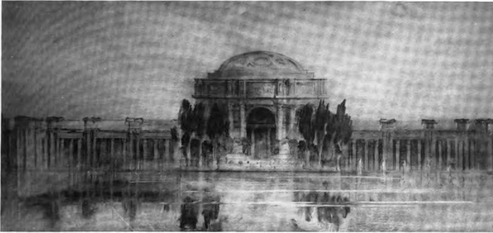
FRONT ELEVATION OF THE FINE ARTS BUILDING, DESIGNED BY MAYBECK
