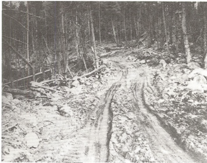
FIGURE 1-17. ROAD BUILT DURING EXPLORATORY ACTIVITY. SOURCE: BLM
