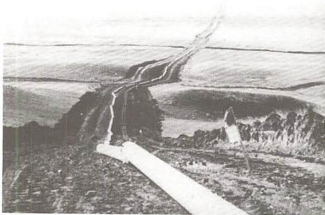
FIGURE 1-28. OIL PIPELINE ROUTE AWAITING ASSEMBLY AND BURIAL.
