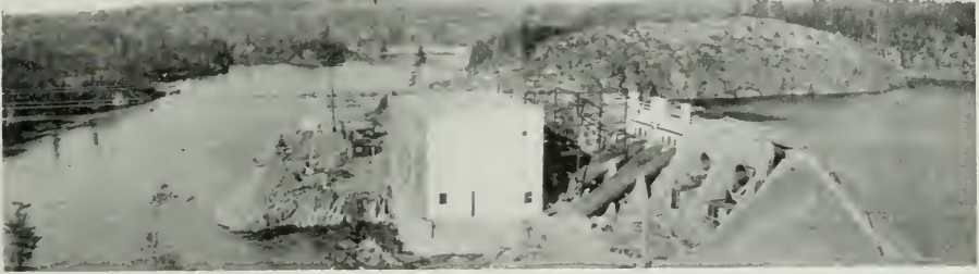
General view, Quinze power plant, Quinze river.
