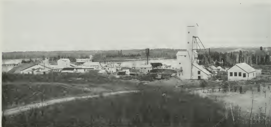
Teck-Hughes gold mine, showing new headframe and hoist-house.
