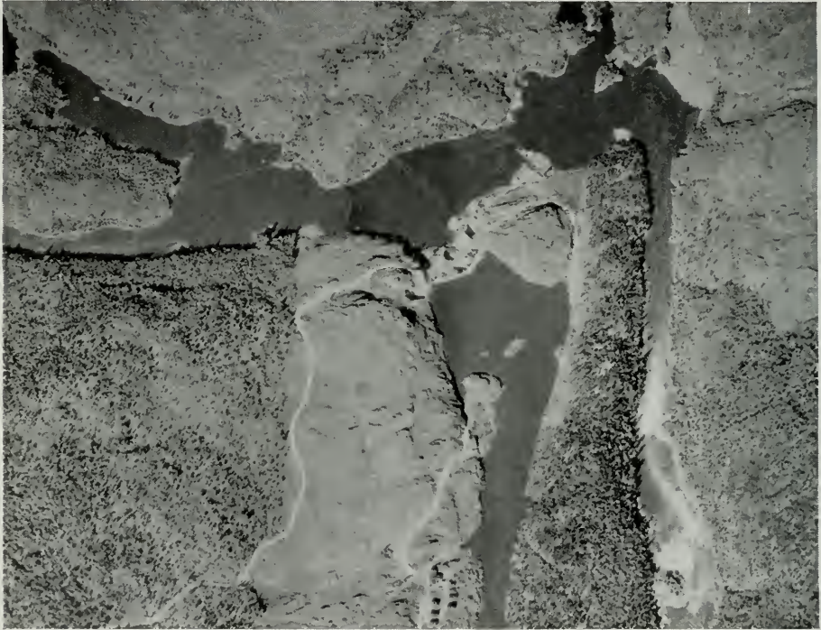
Aerial map of Quinze river power development, reproduced by kind permission of Fairchild Aerial Surveys Co. (of Canada) Ltd., Grand Mere, Quebec.
