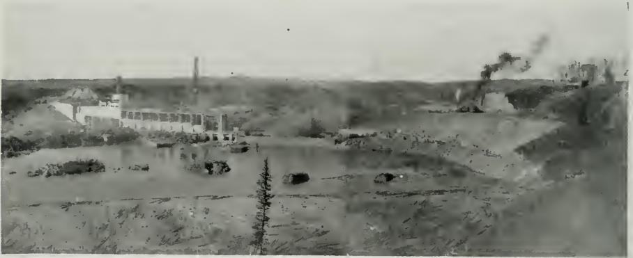
Panorama of power house and dam, water power development at Island Portage on Abitibi river by Hollinger Consolidated Gold Mines, Ltd., Oct. 16, 1924.
