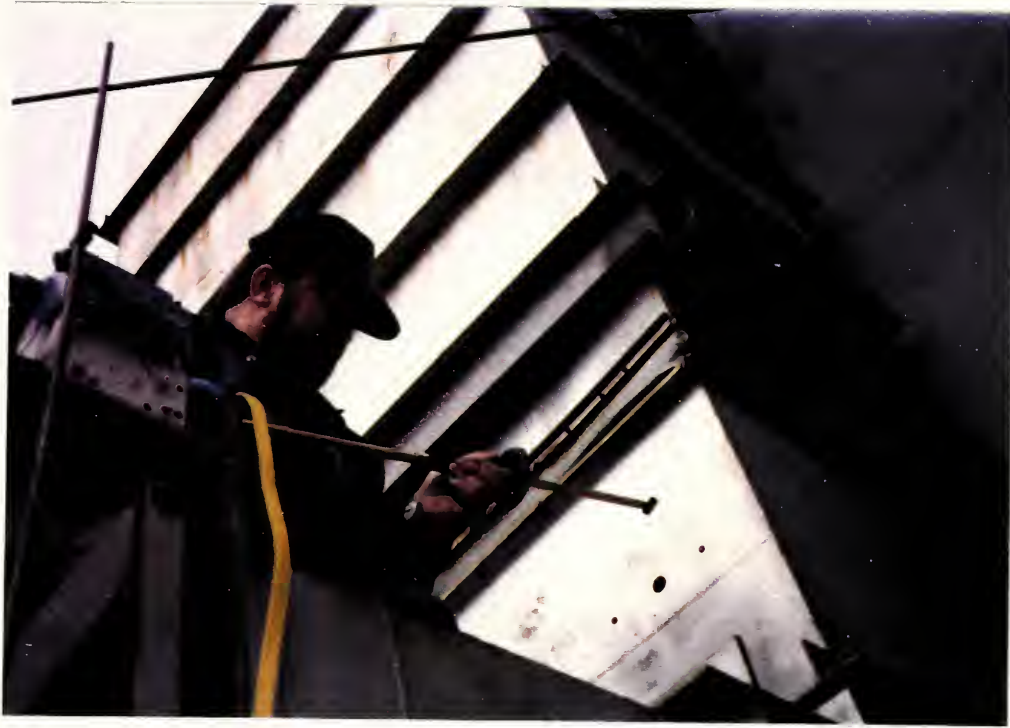
Figure 15A. Typical Hole for Pitot Tube
