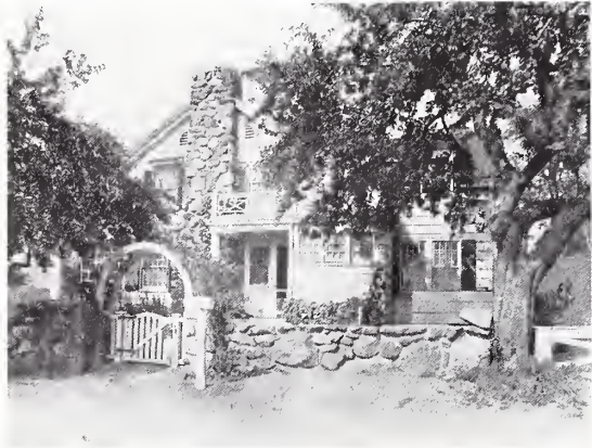
THE SUPERINTENDENT'S COTTAGE
