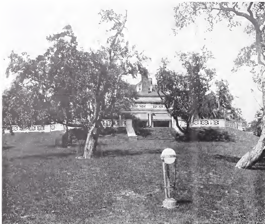
A VIEW FROM THE SOUTH, SHOWING ROAD LAMP, GRASS STEPS, TERRACE, ETC.
