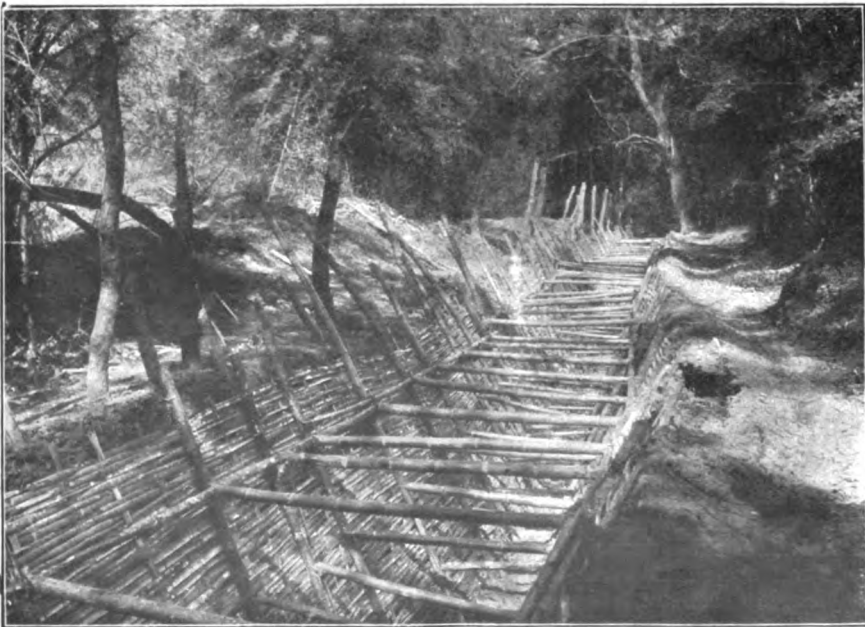
A KEDDAH TRENCH, WITH LINING AND CROSS THWARTS OF BAMBOO TO PREVENT SUBSIDENCE OF THE LOOSE EARTH SIDES. From a Photo.
