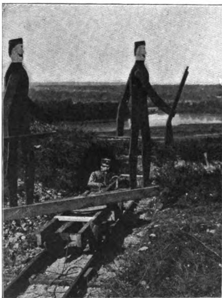
THE RUNNING MEN, SHOWING HOW THEY ARE WORKED FROM THE PIT.
