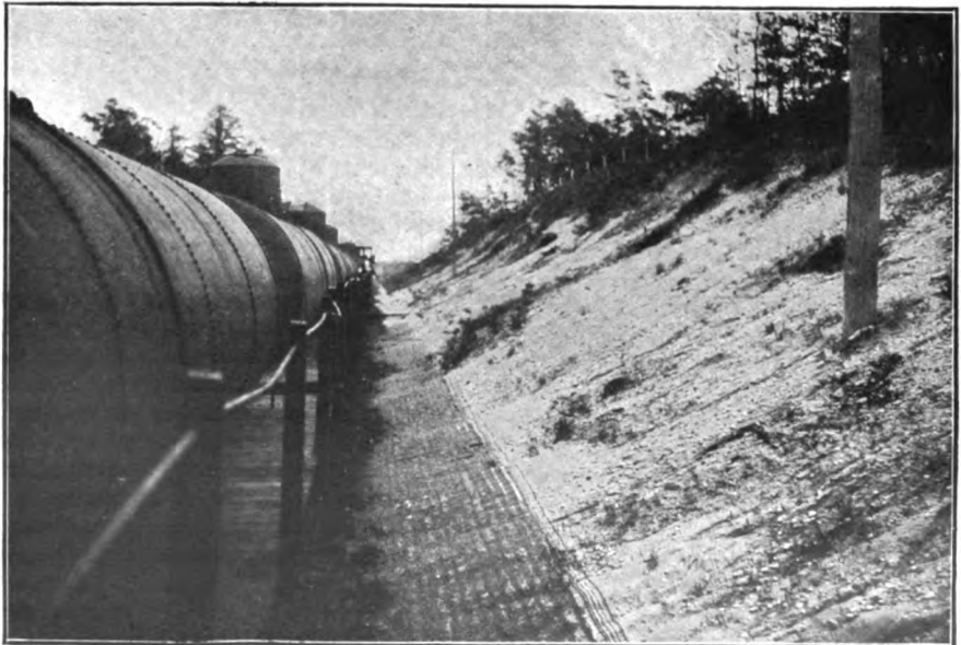
THE TANK-CARS, FILLED WITH OIL, WITH CUTTING, AT SIDE, COVERED WITH OIL.
