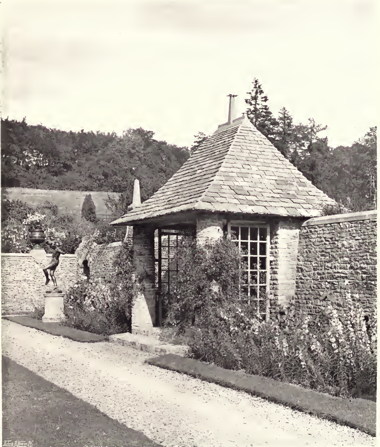
171.—AT NETHERSWELL MANOR. DESIGNED BY MR. E. GUY DAWBER.
