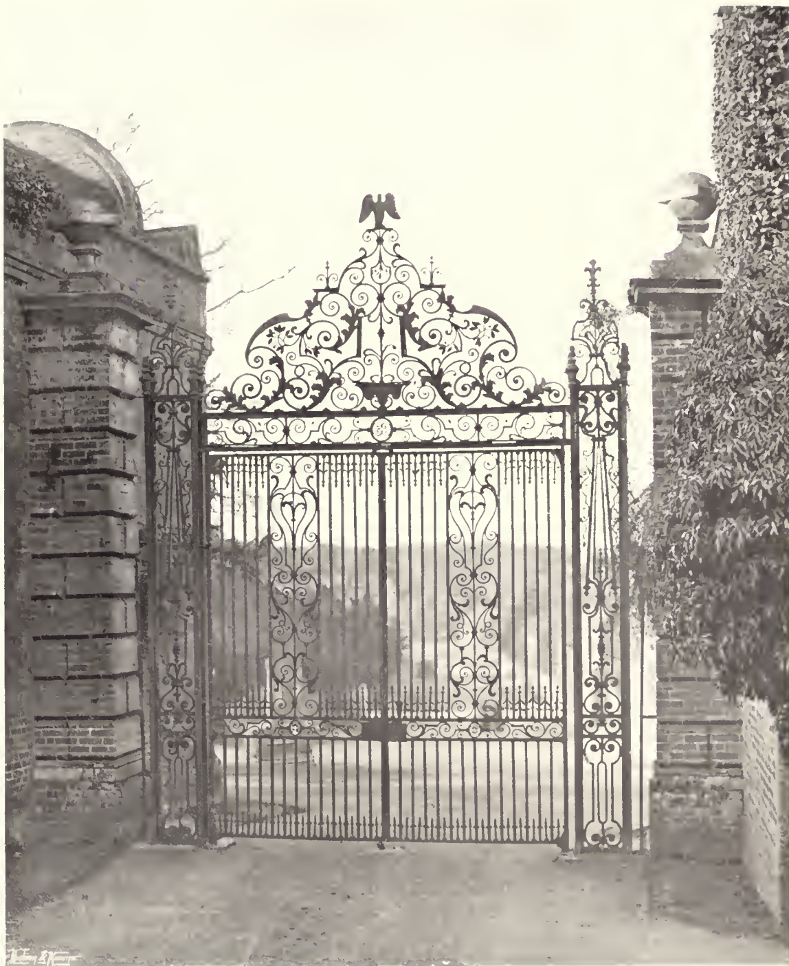
215.—WILLIAM III. GATE AT ALDERMASTON.
