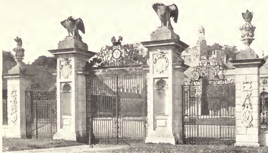
213.—THE FORECOURT GATES TO DRAYTON HOUSE: PROBABLY BY JEAN TIJOU.
