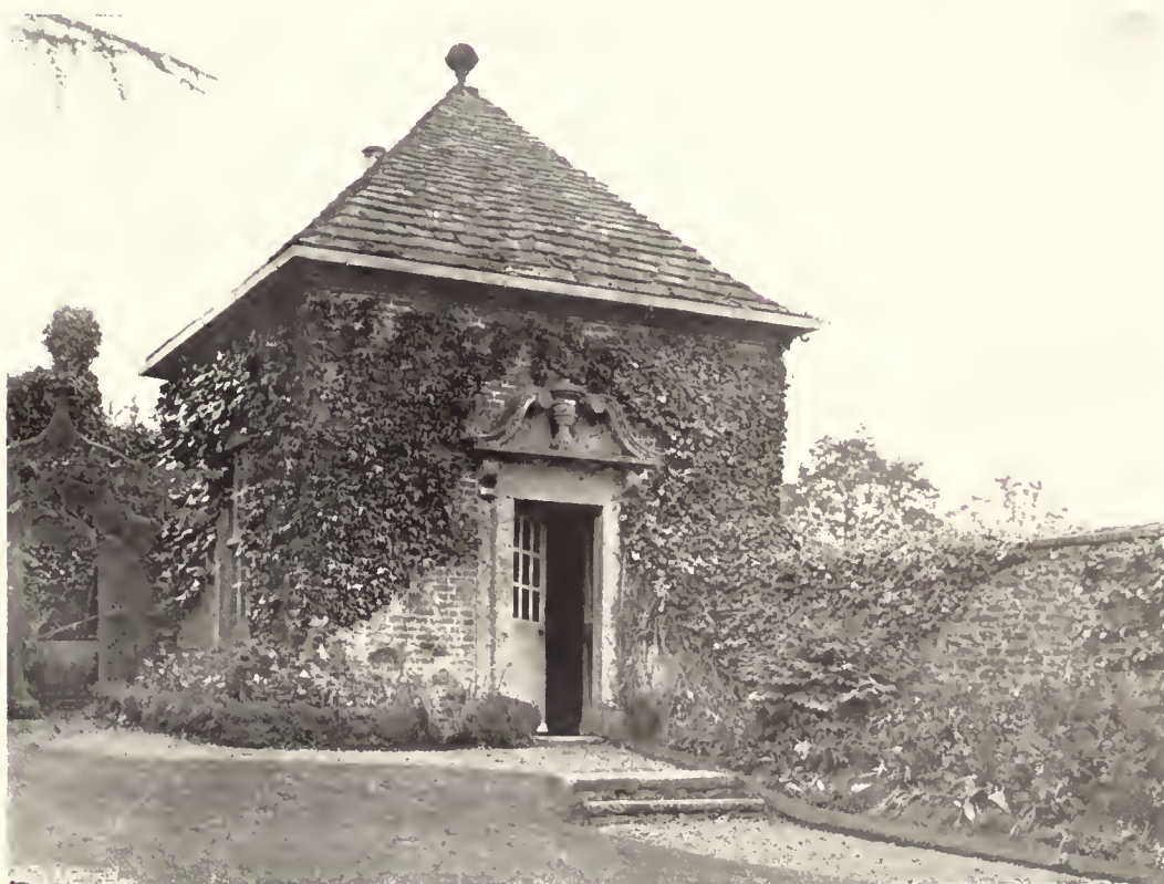
166.—GAZEBO AT BECKINGTON: OF BRICK WITH STONE-TILED ROOF.
