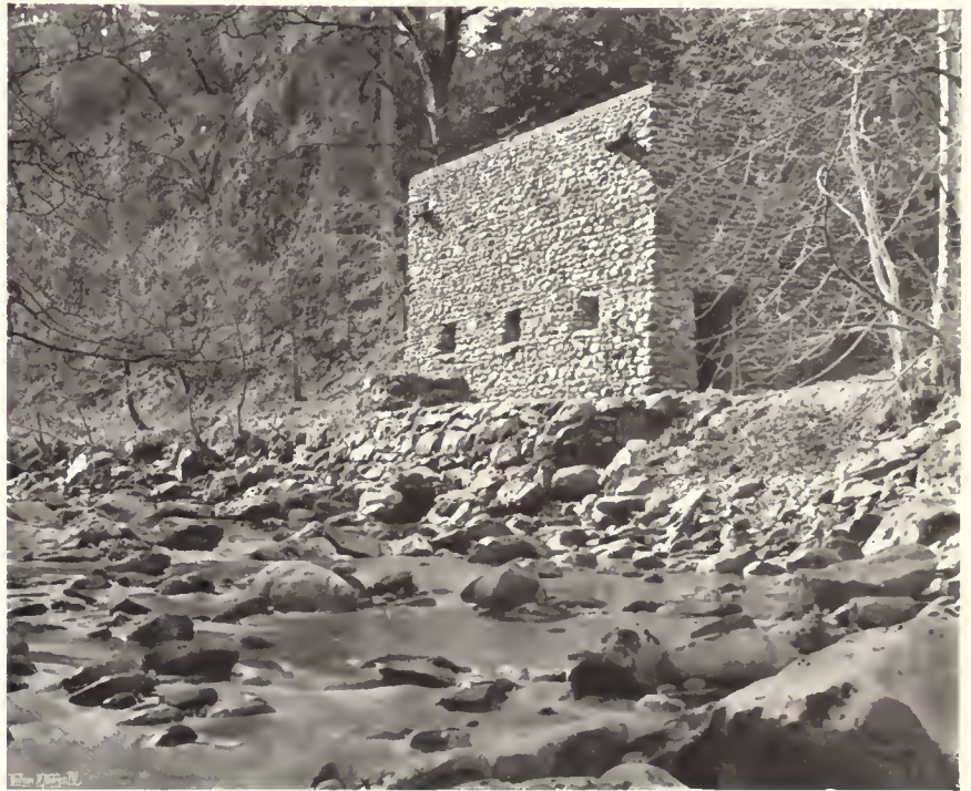
141.—THE POWER-HOUSE AT ARDKINGLAS.
