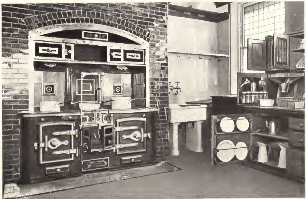
122.—RANGE WITH ROASTING FIRE AND NEW TYPE BATH BOILER
