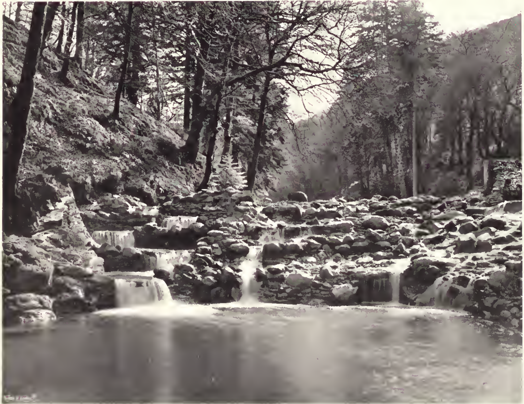
142.—THE DAM AND SALMON LADDER.
