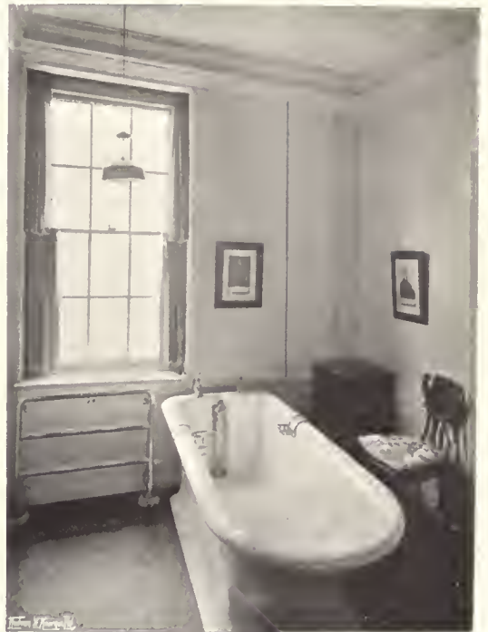
130.—STANDING OUT INTO THE ROOM.
