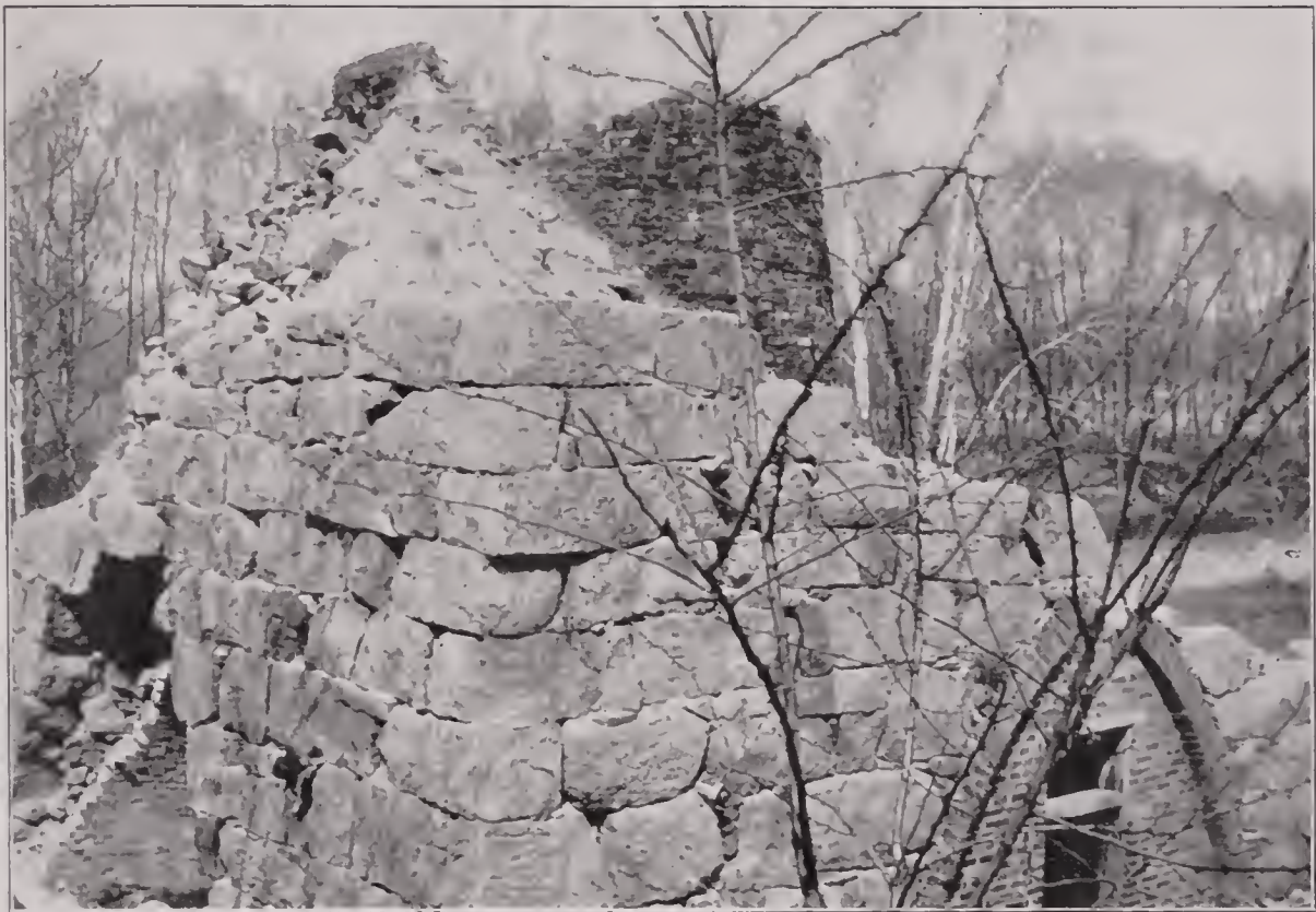
FIG. 1.—RUINS OF ELKRIDGE FURNACE, ELKRIDGE, HOWARD COUNTY.
