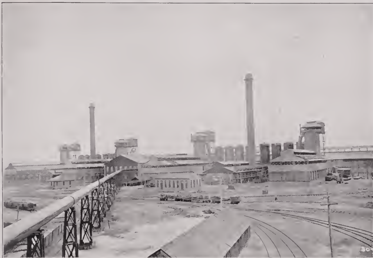
FIG. 1.—BLAST FURNACES, MARYLAND STEEL COMPANY, SPARROWS POINT, BALTIMORE COUNTY.
